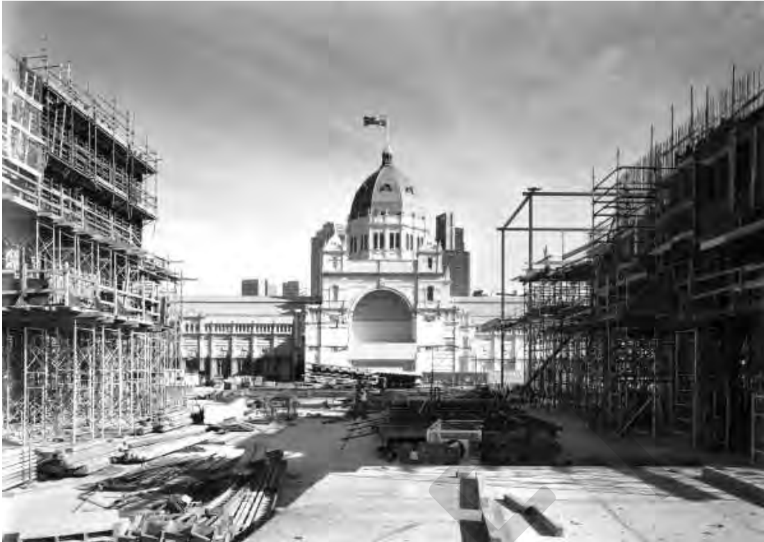
Figure 104 North elevation of the Exhibition Building viewed from the Melbourne Museum construction site, 1998 Source: Picture Collection, State Library of Victoria
