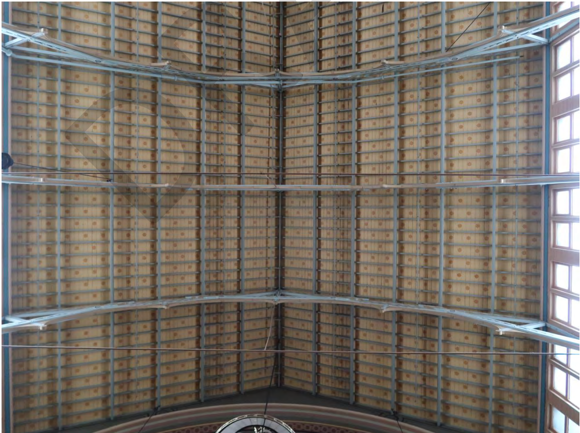
Figure 24 View of the underside of the ceiling and roof structure
