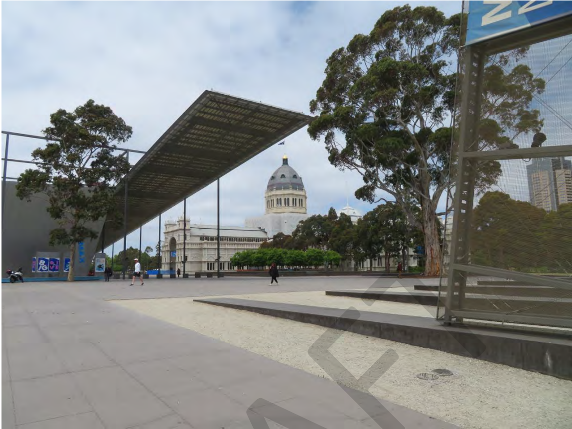
Figure 51 View of the west entry canopy to the Melbourne Museum with the REB behind
