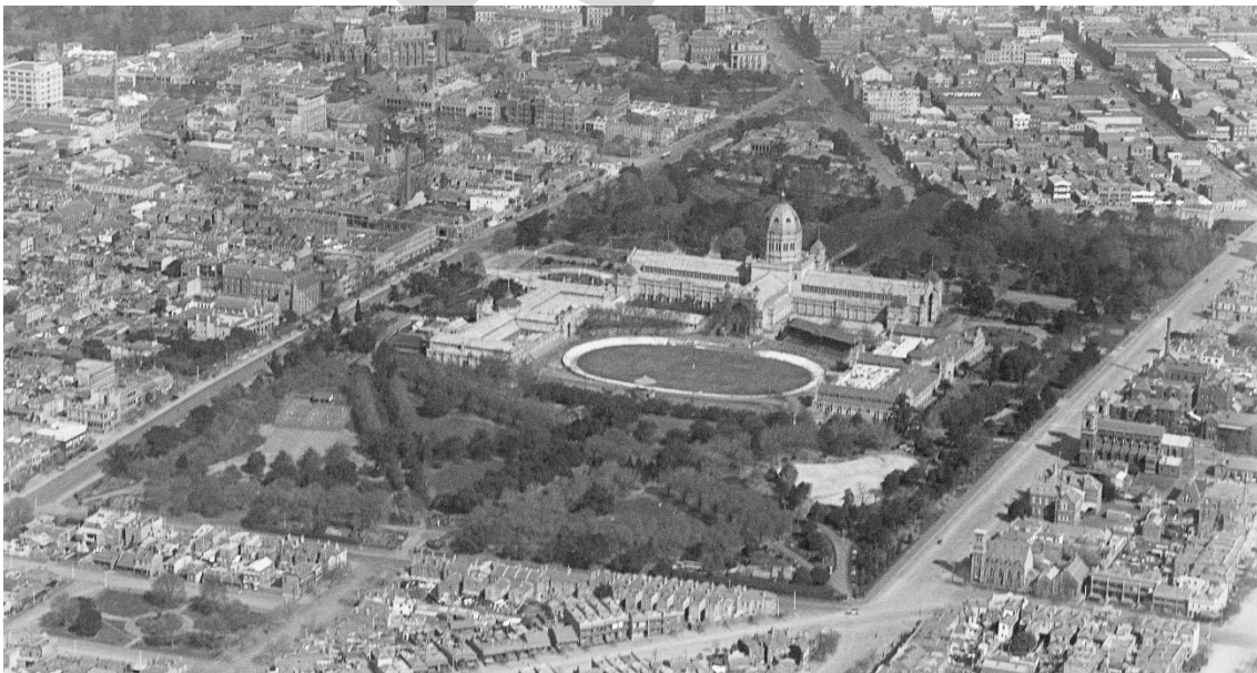
Figure 33 Airspy oblique aerial photograph, c. 1930-48, showing location of tennis courts and children's wading pool in the North Garden Source: H91.160/514, Airspy collection, State Library of Victoria
