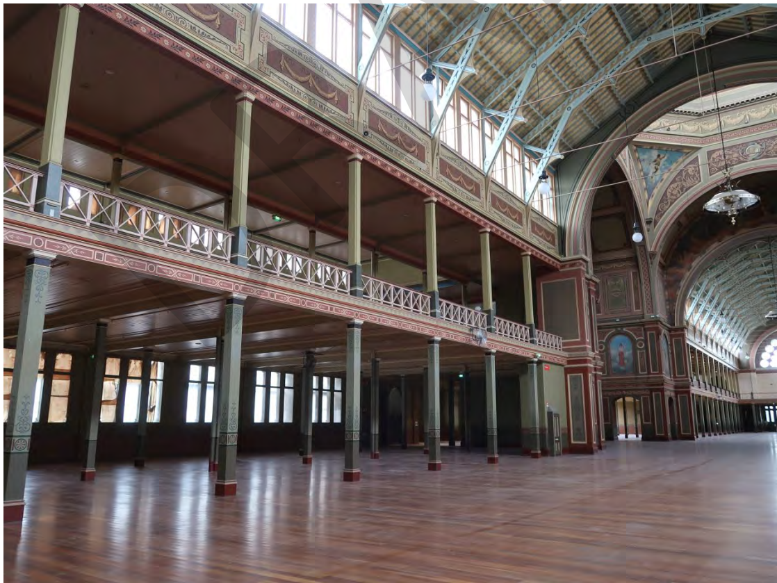
Figure 22 View to the southern side of the east transept; note the timber structural system and the upper clerestory
