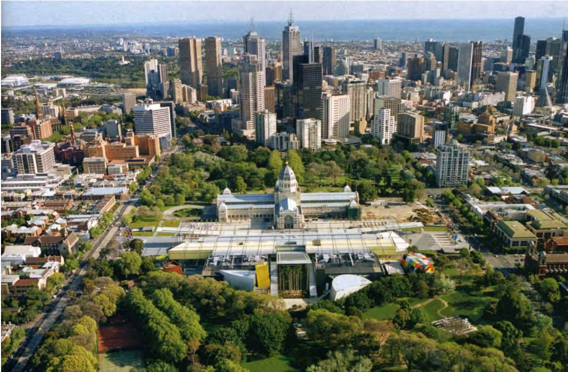
Figure 27 Oblique aerial view from the north of the Exhibition Building, Carlton Gardens and the Melbourne Museum designed by Denton Corker Marshall showing its northern façade entrance aligned with the Exhibition Building's north-south axis, c. 2001 Source: Reproduced from Architecture Australia
