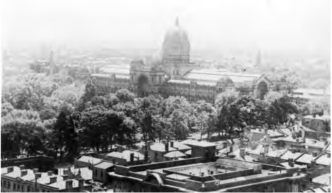
Figure 86 View of Melbourne showing the Exhibition Building, c. 1930. Source: Picture Collection, State Library of Victoria
