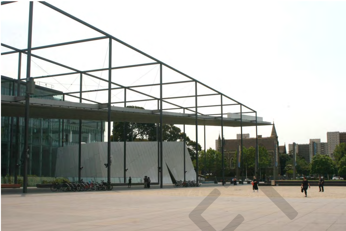
Figure 53 View east-northeast across the Museum Plaza towards the entry blades / loggia
