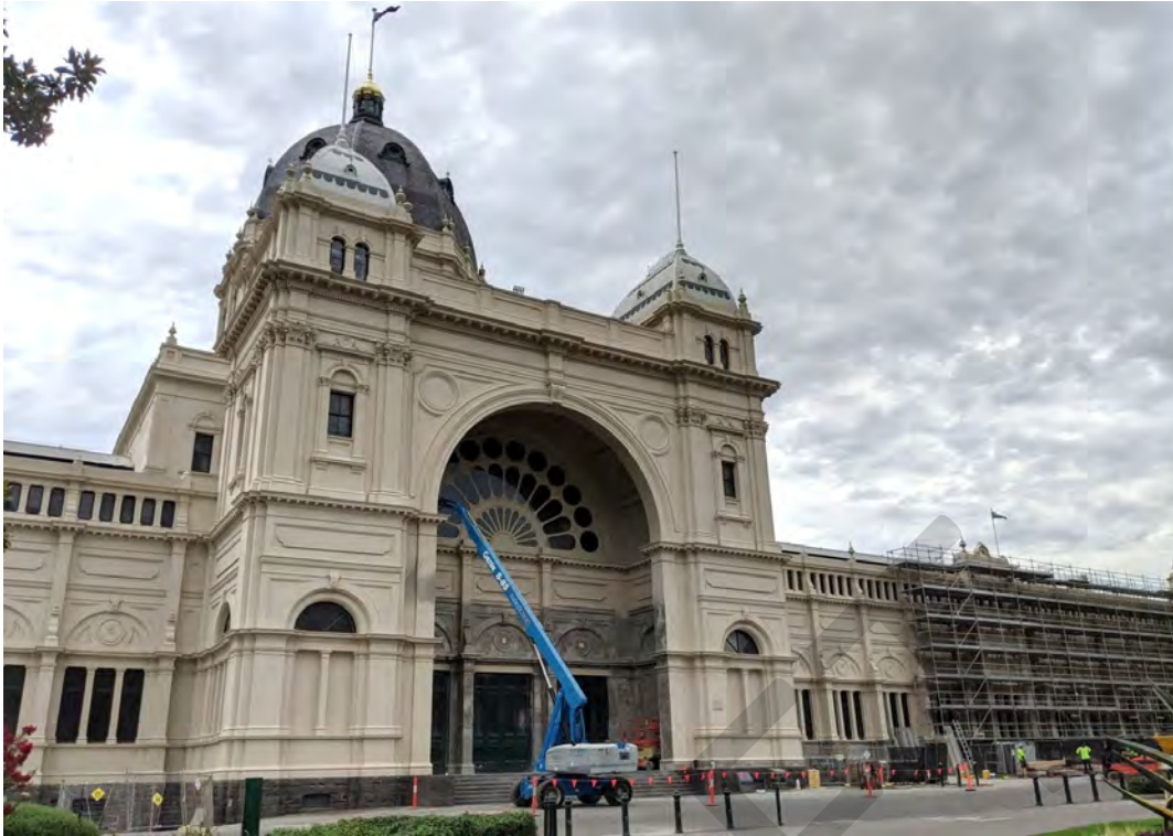
Figure 4 South elevation, central porch; note repair works underway (2020)
