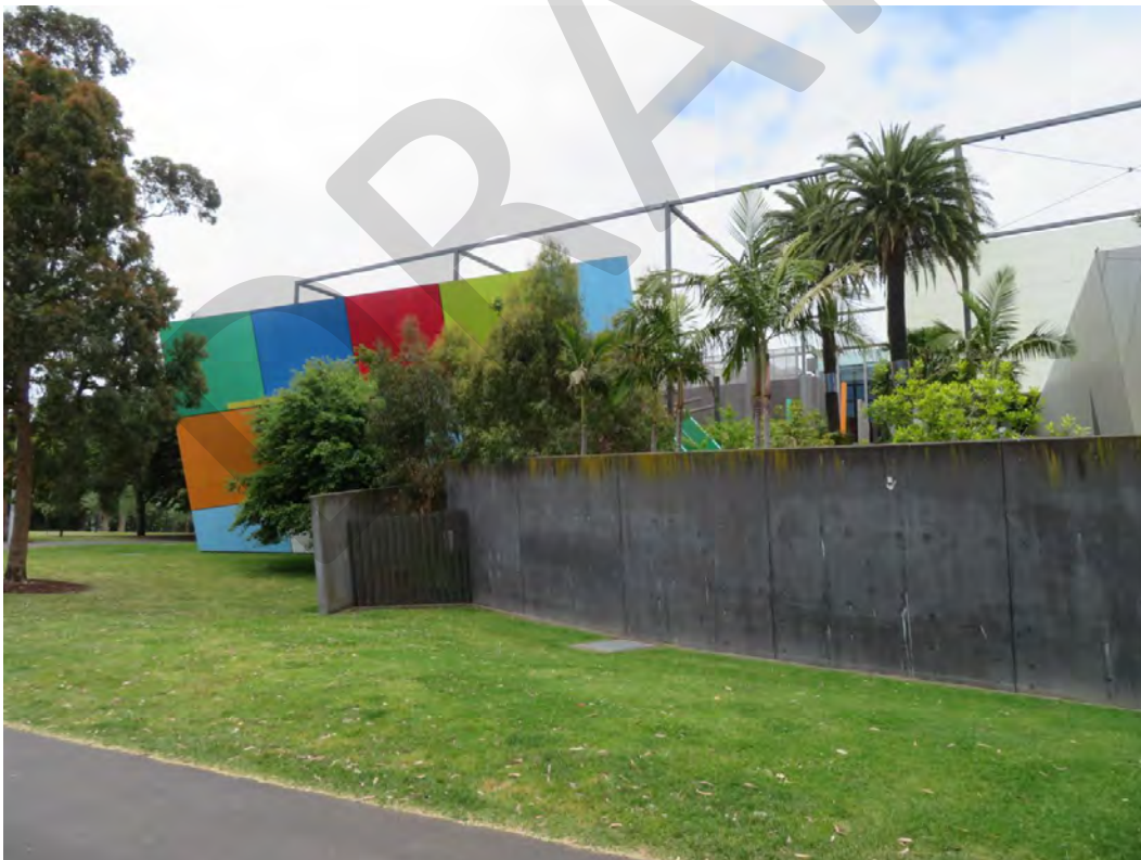
Figure 48 View of Melbourne Museum from the western edge of the Carlton Gardens; note the grid structure over the top of the individual volumes and the colourful Children’s Museum
