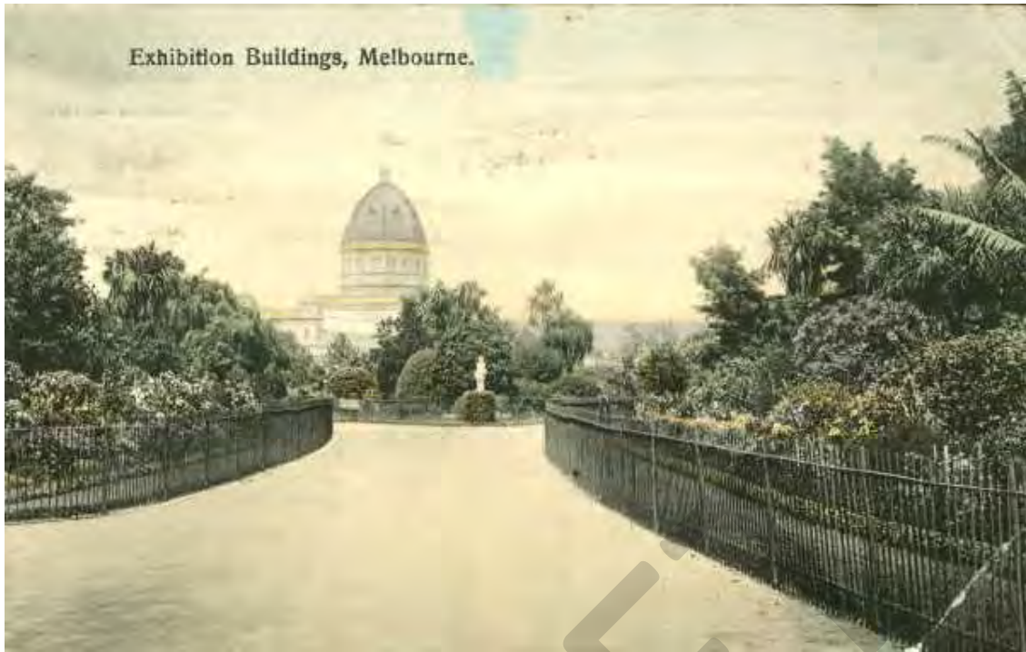
Figure 68 Carlton Gardens, c. 1905, showing a high metal palisade fence separating the wide path from the formal, deeply layered garden beds. Source: Picture Collection, State Library of Victoria
