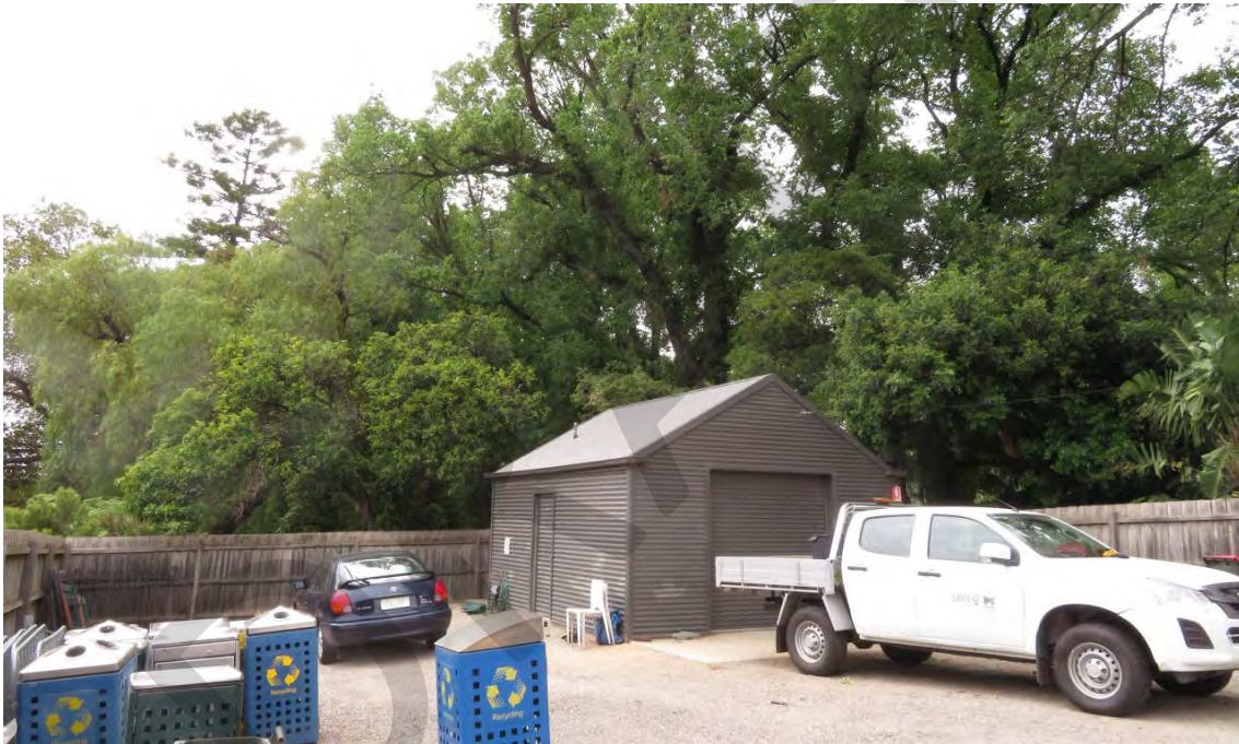
Figure 92 Works depot east of Curator's Lodge
