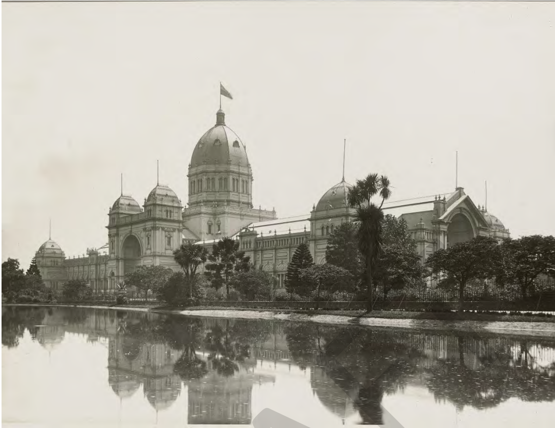
Figure 84 View Exhibition Building c. 1926 Source: Picture Collection, State Library of Victoria
