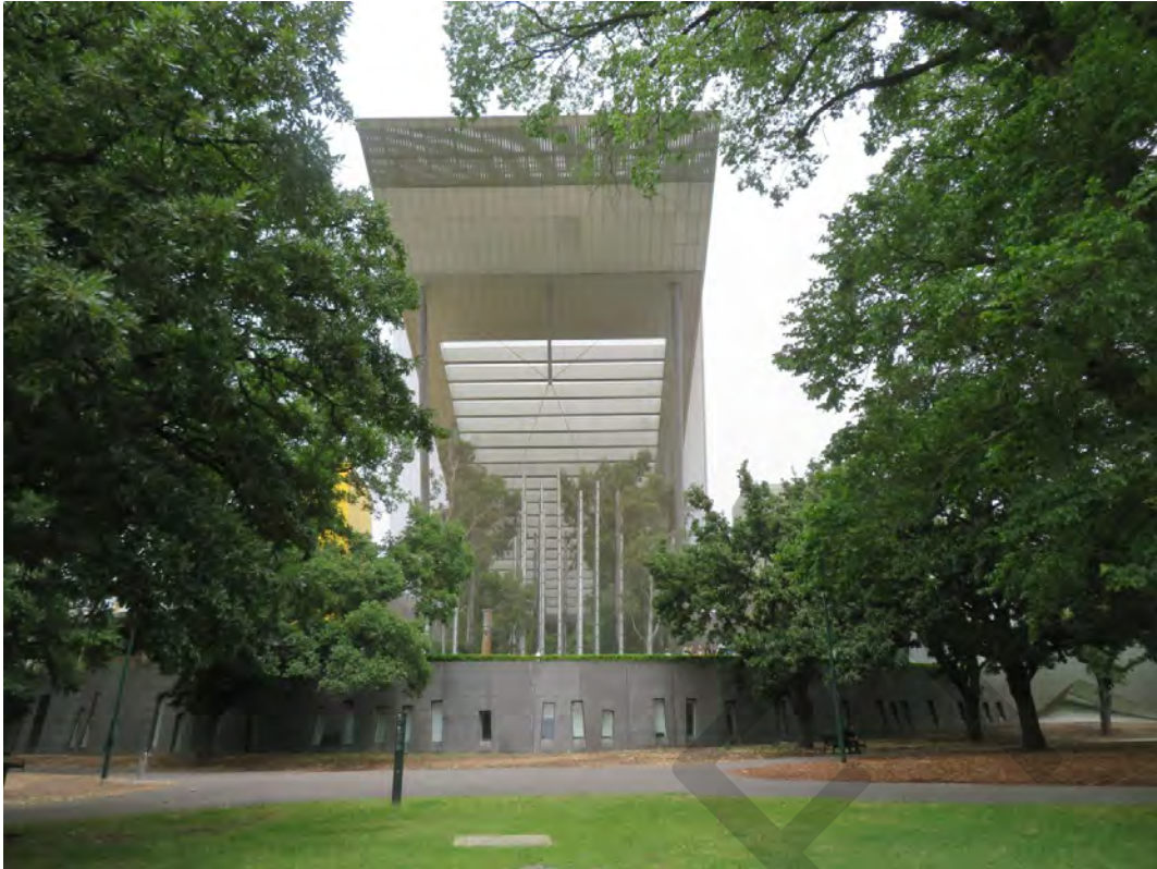
Figure 49 View of the north wall of the Museum and blade roof and Forest Garden from the Carlton Gardens
