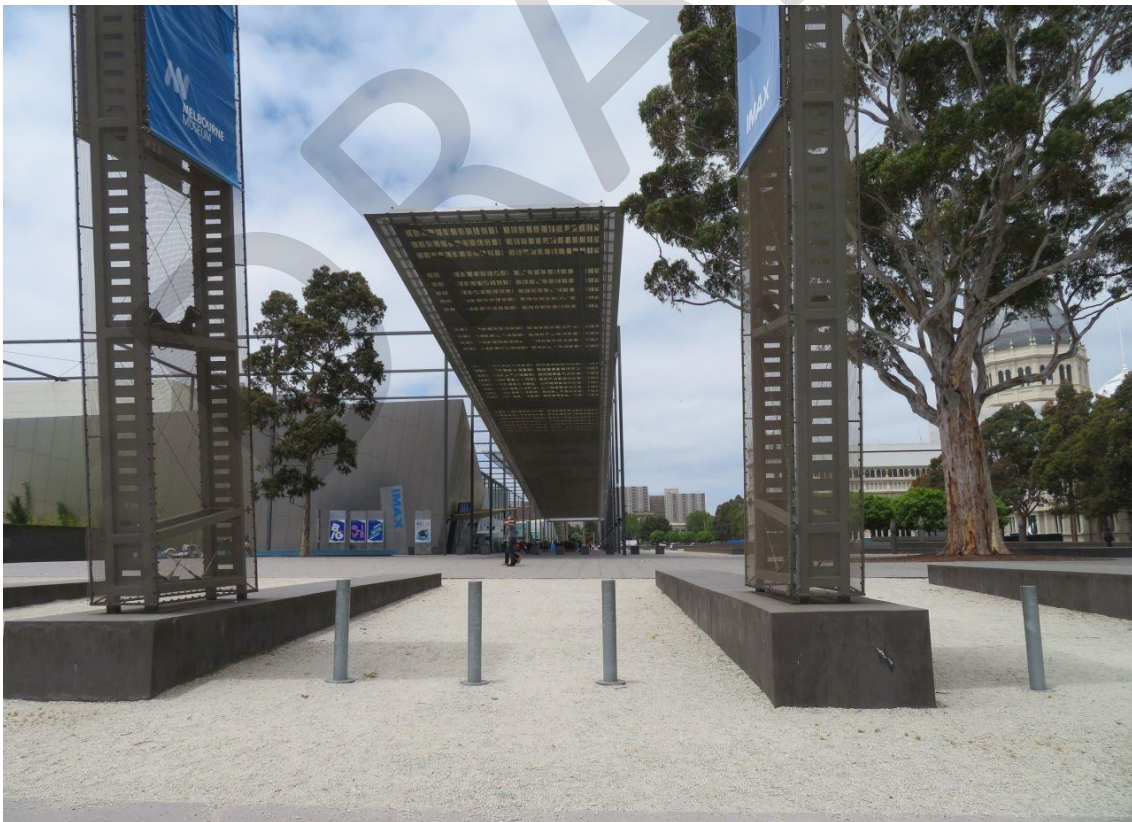
Figure 16 View of the Melbourne Museum and Museum Plaza from Rathdowne Street
