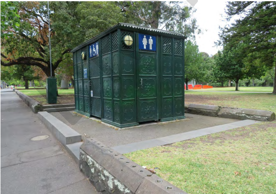
Figure 96 North toilet facilities, viewed from the south-west
