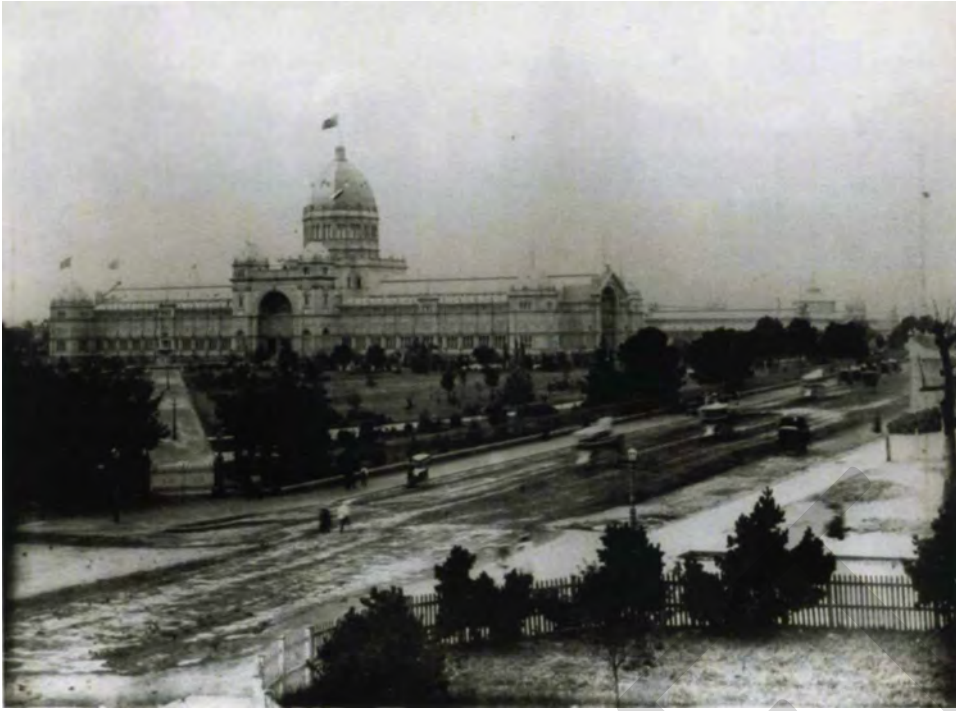
Figure 28 View of the Nicholson Street side of the Carlton Gardens seen from Victoria Parade, c. 1881, showing the then new iron gates and railing Source: Reproduced from Melbourne's Historic Public Gardens: A Management and Conservation Guide
