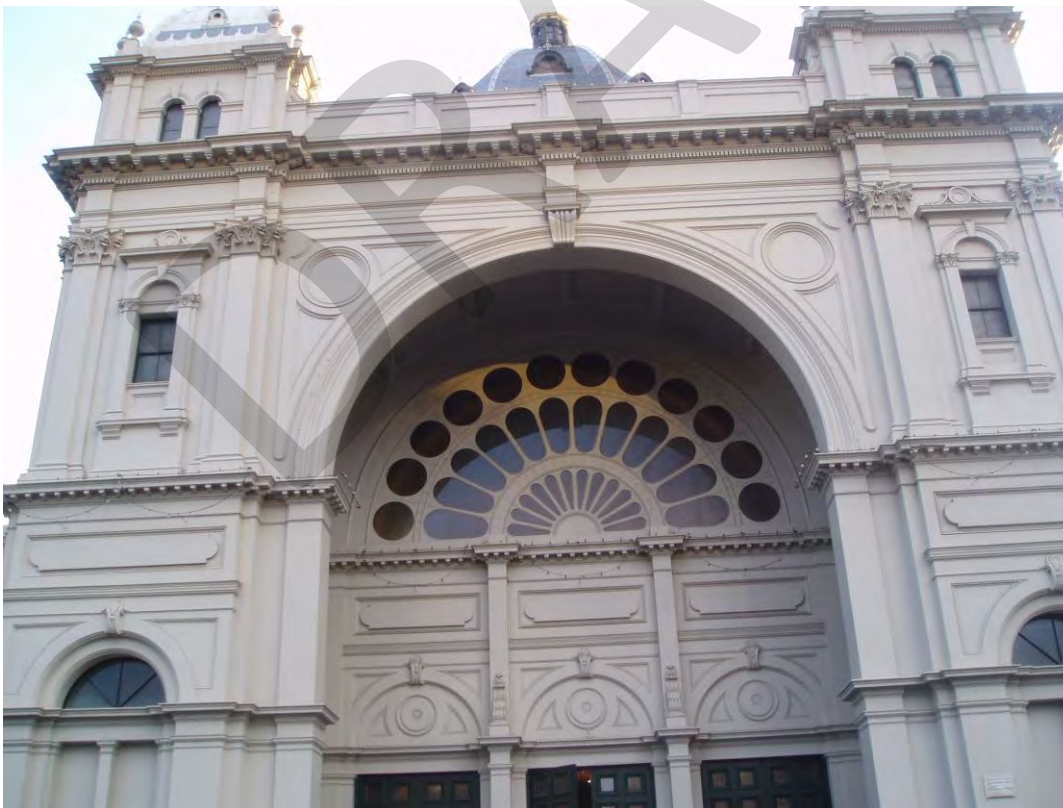
Figure 5 Fanlight over the main porch entrance in the south elevation, prior to recent restoration works
