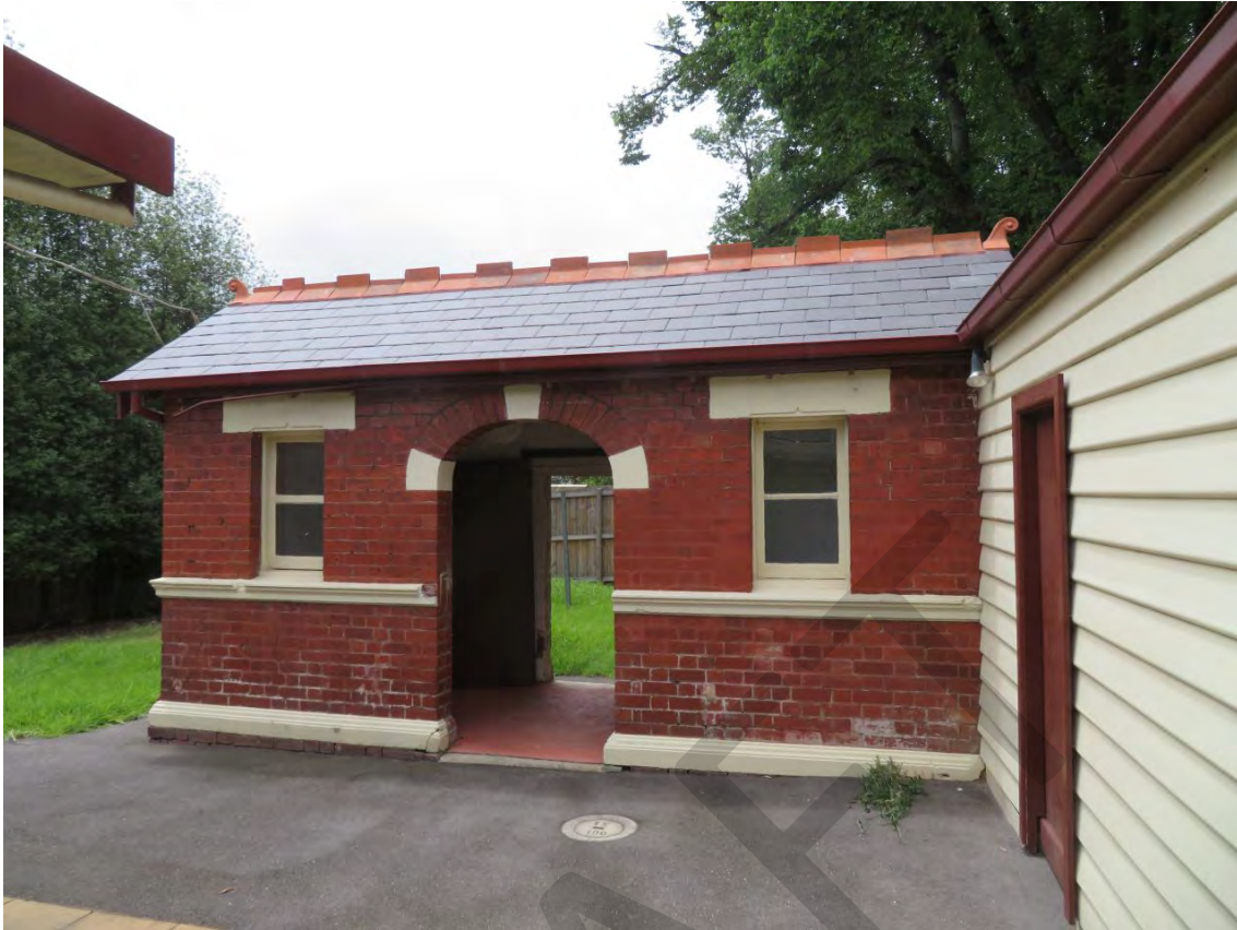
Figure 82 West façade of the rear outbuilding, weatherboard garage at right
