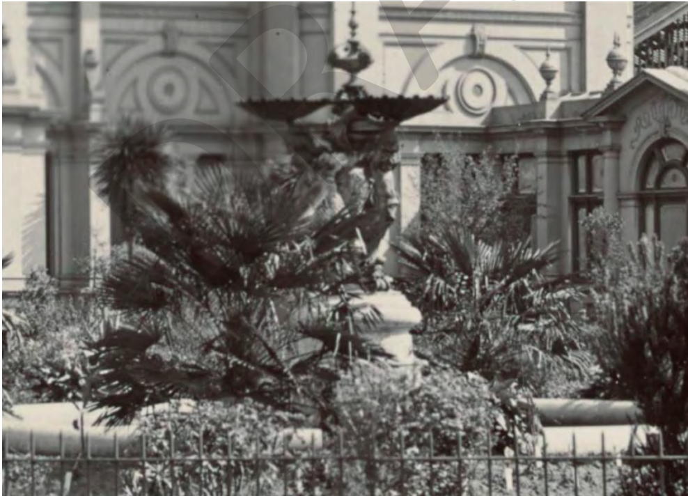
Figure 21 French Fountain c. 1885-90. Note the pedestal base and basin are rendered brickwork with what appears in the black and white photograph to be a light stone coloured finish. The pedestal base is elaborately moulded. The finial to the fountain is in place. Source: Detail of H84.202/20, Picture Collection, State Library of Victoria
