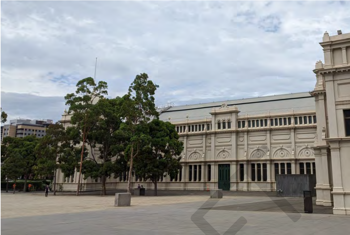
Figure 11 North elevation, eastern nave
