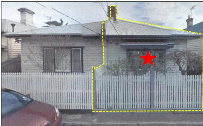
The subject site when viewed from Canterbury Street (DX Architects, August 2019)
