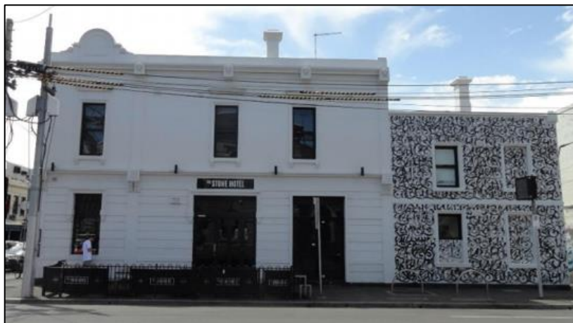
Figure 13 - Chimneys visible from Johnston Street
