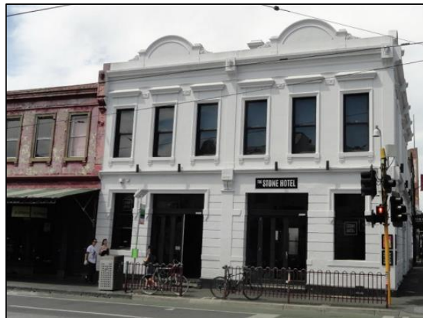
Figure 11 – Chimney partially visible from Brunswick Street
