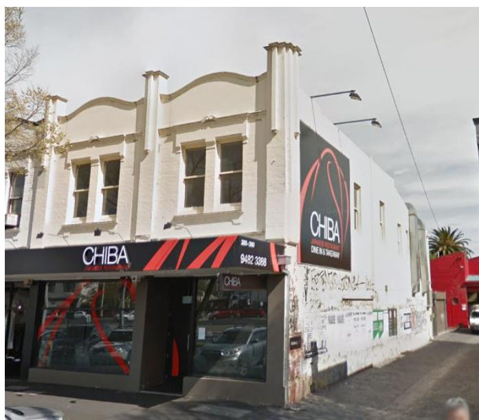
Figure 4 – Subject site viewed from Queens Parade (Google Streetview Oct 2016)
