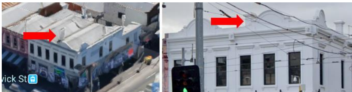
Figure 12 - Brunswick Street Chimney
