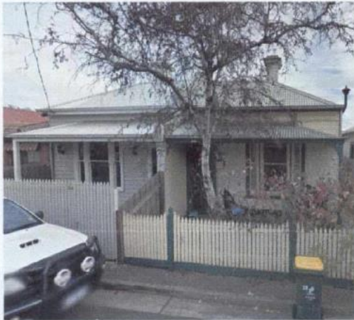
....no. 34 & 32 canterbury street..
