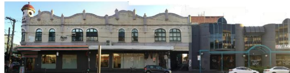
NORTHERN ELEVATION OF JOHNSTON ST
