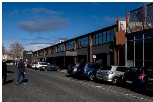
Figure 3: Existing Conditions Griffiths Street
