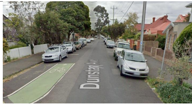
Dunstan Avenue, Brunswick – Parking on both sides of the road.
