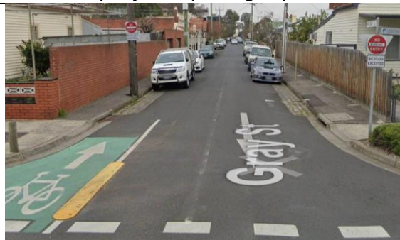
Gray Street, Brunswick – Parking on both sides of the road.
