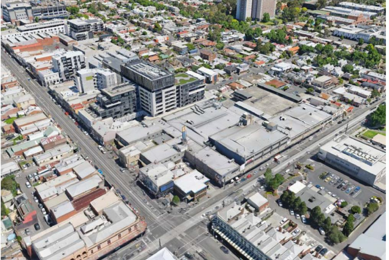
(Looking north – west along Bridge Road)
