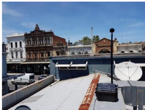
Figure 3 Location of the Noise Logger on the Roof of 171 Swan Street
