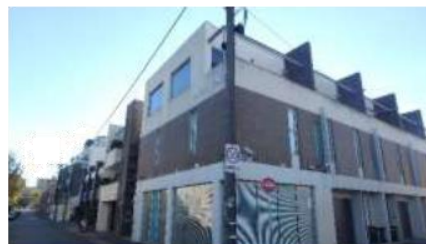
View of 3 storey apartment at 71-73 Rose Street
