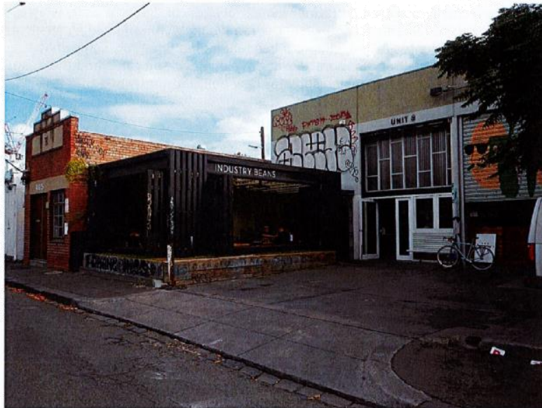
Figure 2 The south part of the site: the temporary structure (black) on the site will also be demolished. Note the small inter-War commercial building (artist's studio) abutting the south boundary. There are single and double storey heritage dwellings beyond (south) the site in Fitzroy Street.
