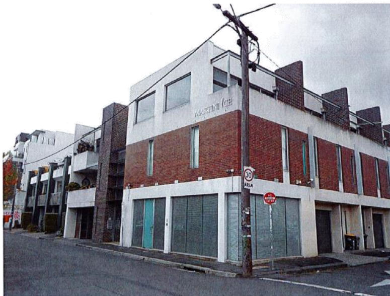
Figure 8 No. 71-73 Rose Street, a 3 storey apartment building on the north-west corner of Fitzroy and Rose Streets opposite the subject site.
