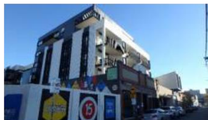
View of 46-52 Rose Street to west (6 storeys)
