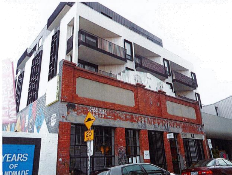
Figure 6 No. 46-52 Rose Street: a 6 storey apartment building retained behind a former industrial façade.
