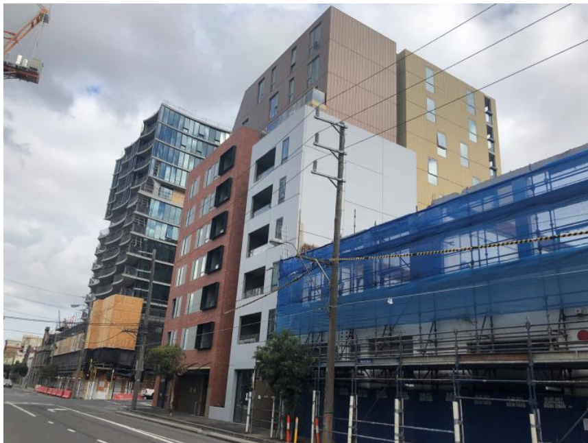
Figure 14: 73-77 Wellington Street, with 61-71 Wellington Street behind
