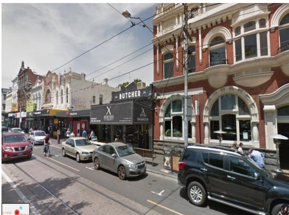
*Figure 6: Individually significant building on the opposite side of Swan Street. Google Maps Nov 2017
