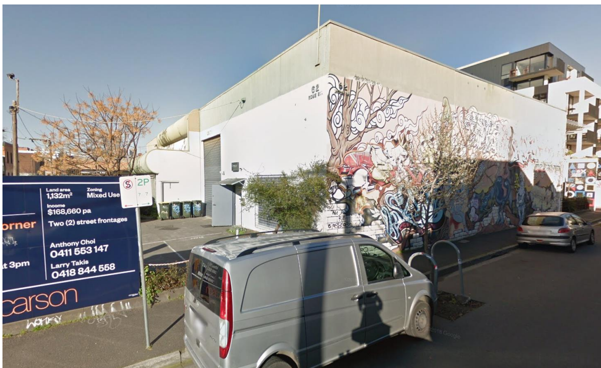
Figure 4: subject site from Rose Street
