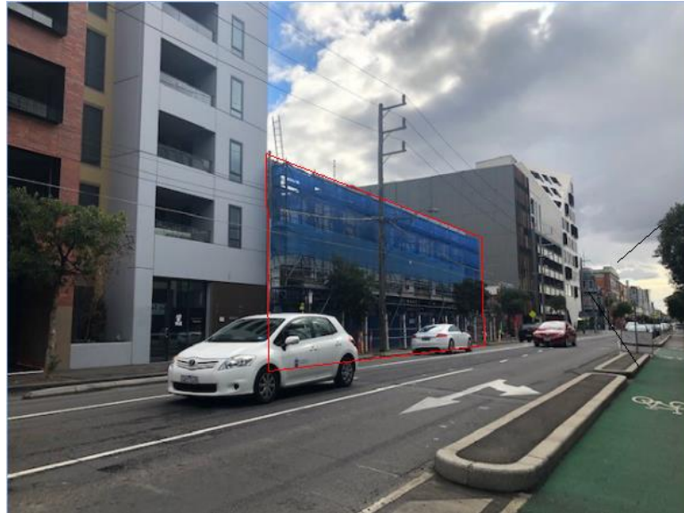
Figure 5: subject site taken 15 June 2019
