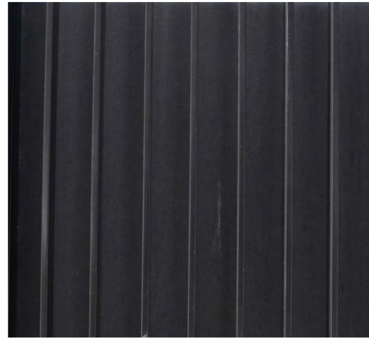
Metal cladding to service locations - solid metal panel, dark grey finish - FT19
