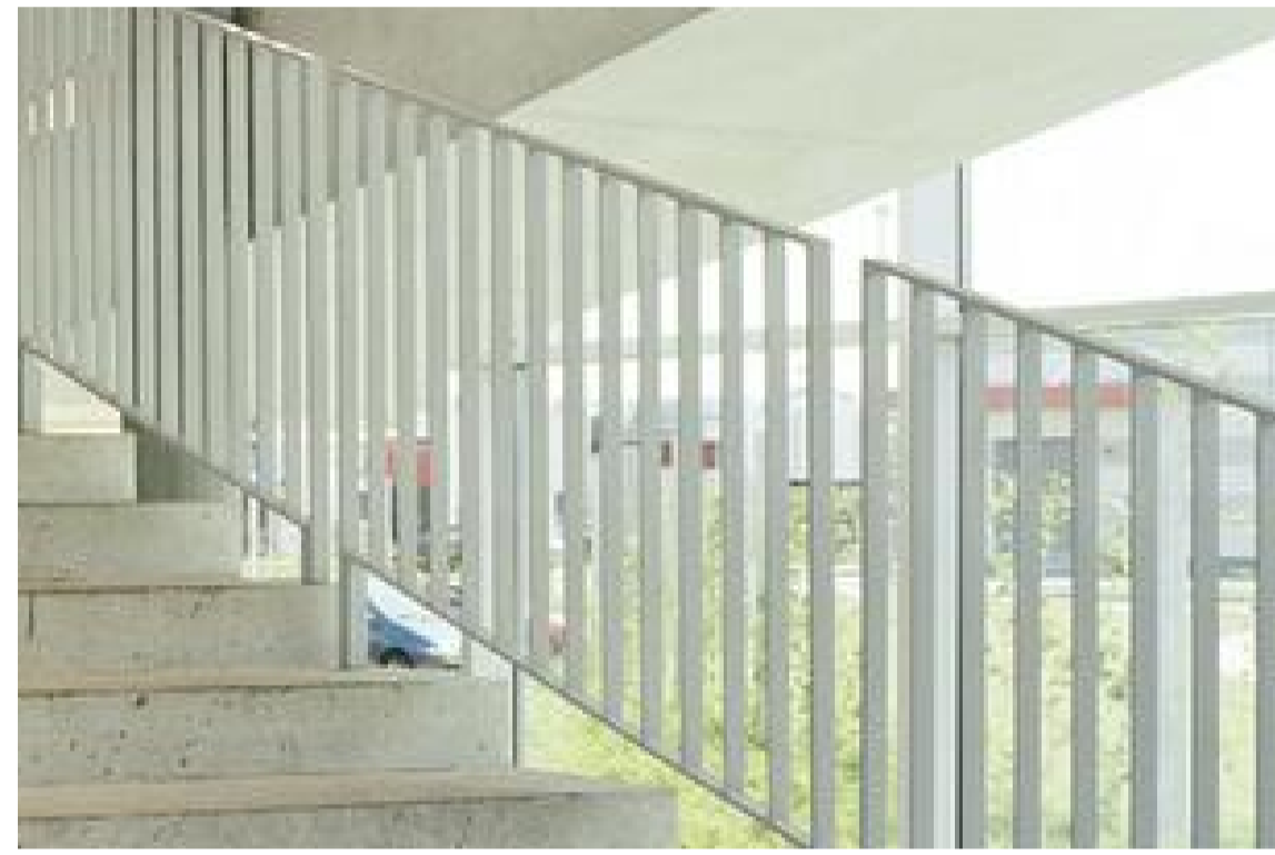
MTL02 - VERTICAL METAL BALUSTRADE
