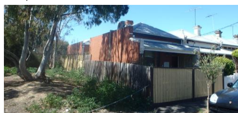
South-west – council reserve, vacant parcel of land and a row of single storey Victorian terrace houses
