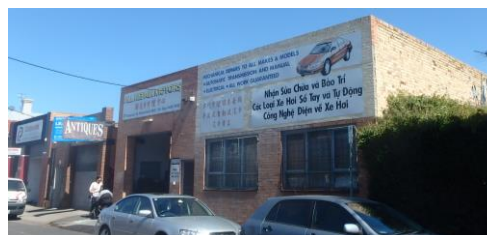
South-east – single storey industrial building at 17 Thompson Street
