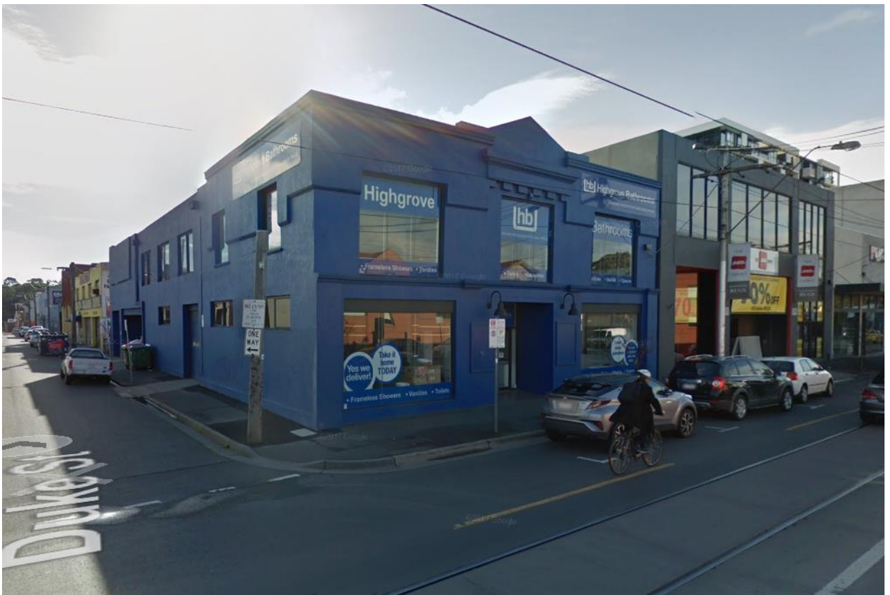
Image 1: The Subject site viewed from Victoria Street (July 2017)
