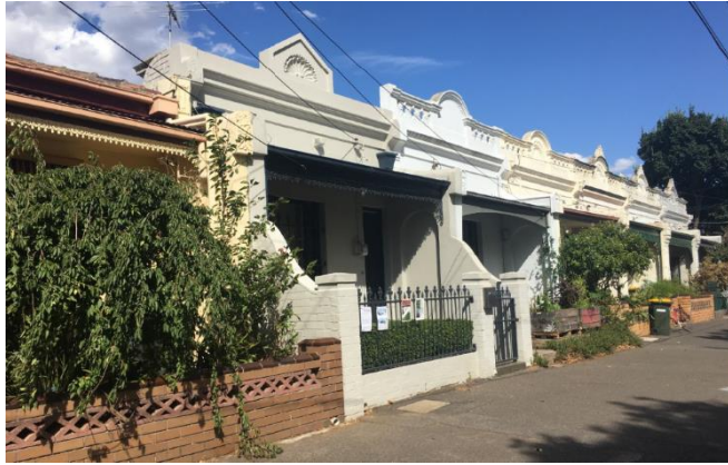
Figure 4: View south along Grant Street (Officer Photo)
