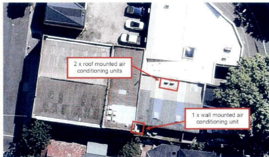
Figure 5: Aerial Photograph Identifying Existing Mechanical Services Equipment
