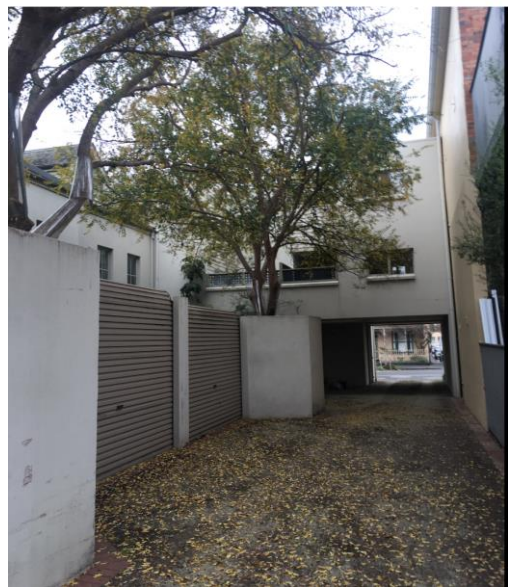
Figure 13: E-1 with building over (Source: officer photos)
