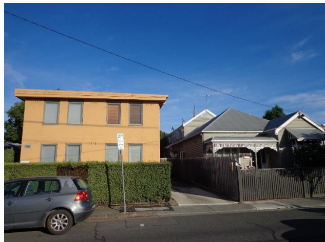
Block of walk-up flats further south
