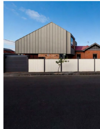
STANDING SEAM CLADDING & ROOF
