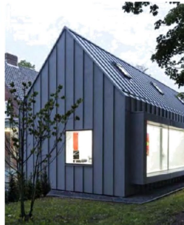
STANDING SEAM CLADDING & ROOF
