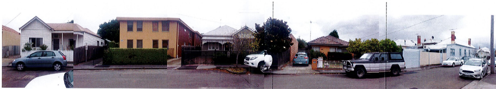
110 Mary St 1 STOREY RES LANEWAY 108 Mary St 2 STOREY MULTI RES 106 Mary St 2 STOREY RES SUBJECT SITE No. 104 MARY ST 28 Mallesov St 1 STOREY RES
