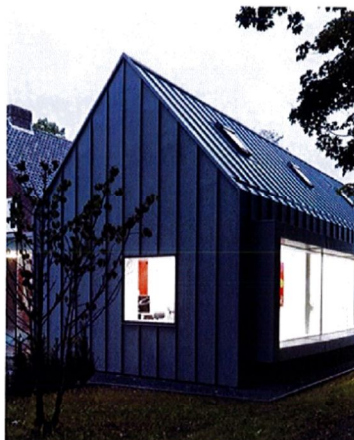
STANDING SEAM CLADDING & ROOF
