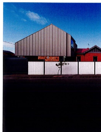
STANDING SEAM CLADDING & ROOF
