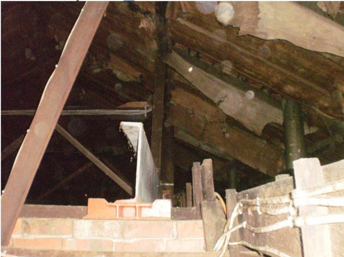
Strengthening beam to roof framing above Hall (viewed looking South).
