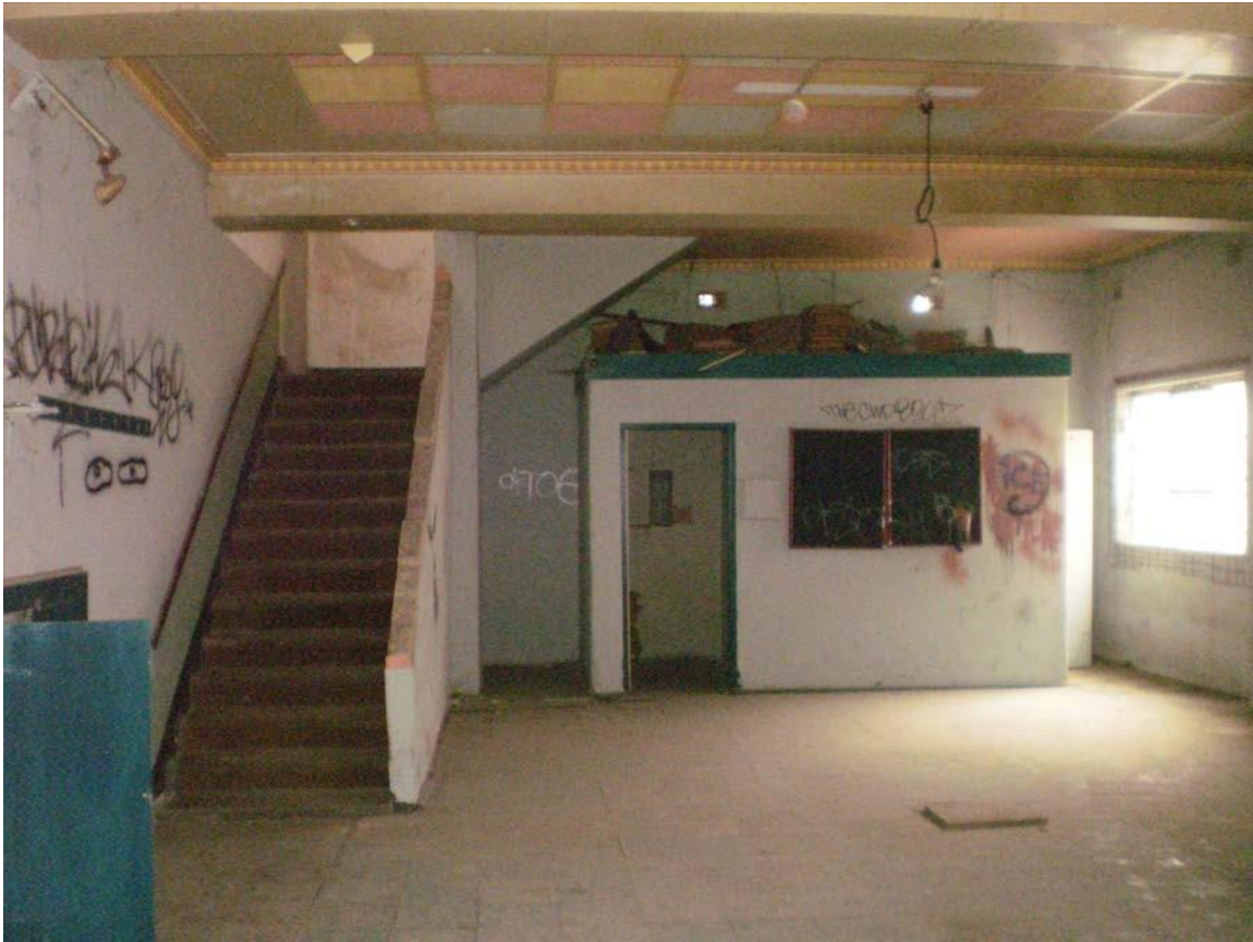
Photo 18: Room 11 viewed looking North. Concrete stair at left.
