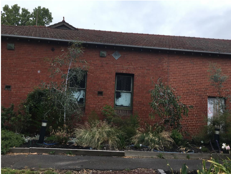
Photo 9: South wall reconstructed. Tie backs within the brickwork restraining wall.
