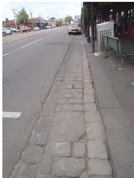
Figure 4.8 : Bluestone channel on east side of Nicholson Street, facing north.
