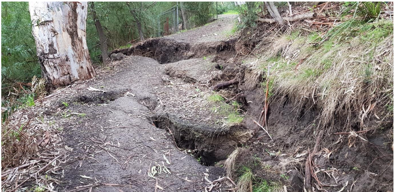
Figure 18. Tree collapse site
