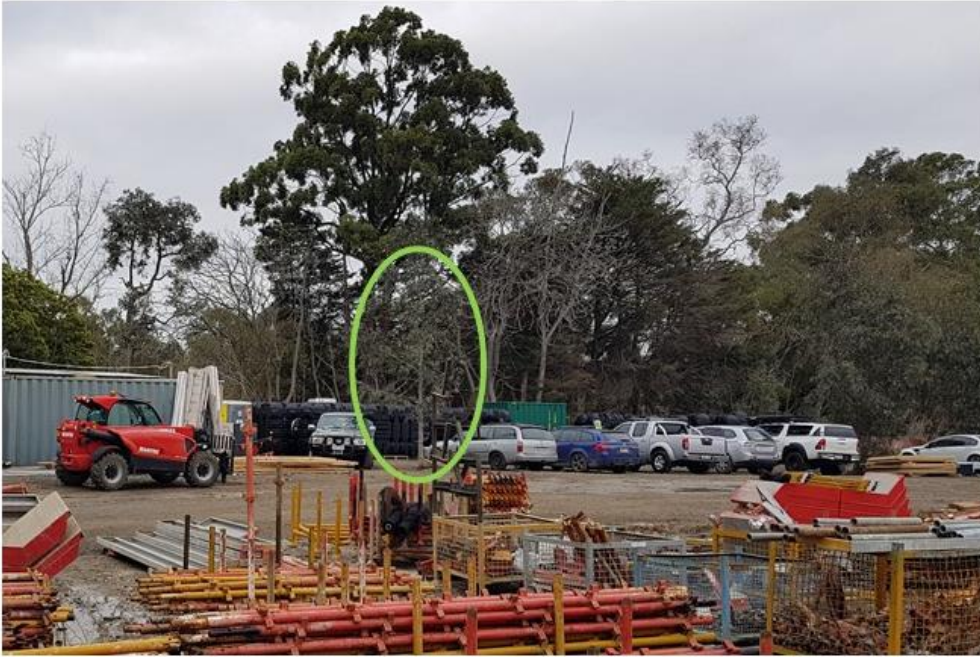
Figure 16: Juvenile tree in carpark - old logistics hardstand
