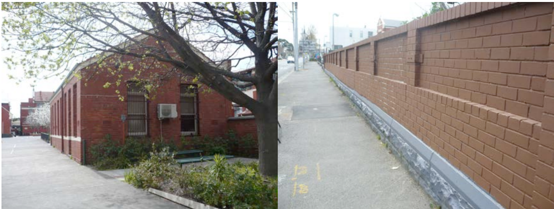
At left, outbuilding at rear of Presbytery. At right, brick fence with original (c.1911) bluestone base.
