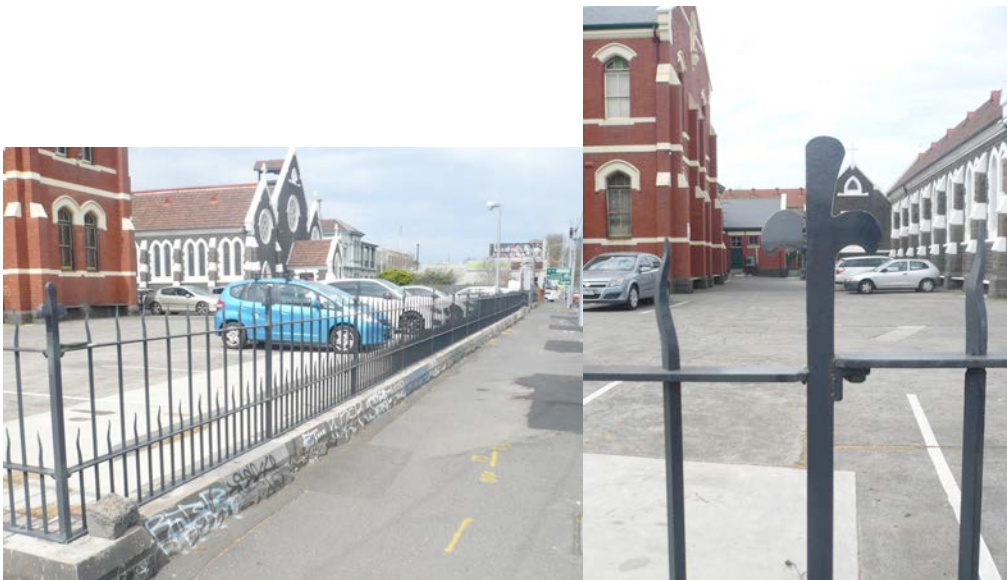
At left, showing the original (c.1911) bluestone base and the recently constructed reproduction iron fence that replaced the original brick wall. At right, showing the juncture between the original fence in front of the church and the reproduction fence in front of the 1897 school.
