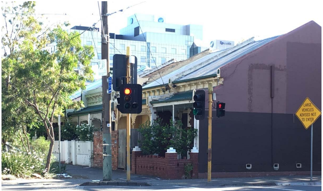
Figure 3. Richmond (terrace row with single roof form, narrow frontages, minimal setbacks on crowded street setting).
