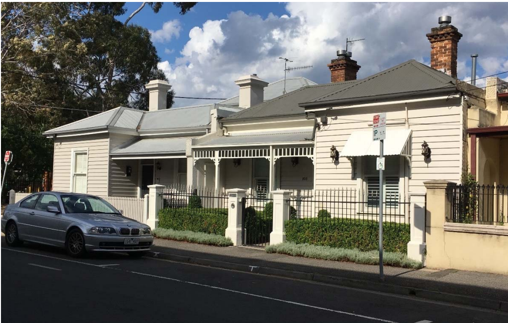
Figure 5. Richmond (wide frontages, minimal setback, semi detached, double fronted houses, wide street).
