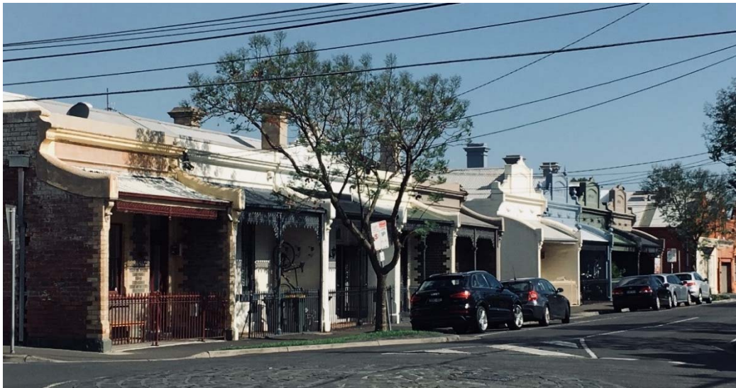
Figure 1. Richmond (typical terrace row with narrow street frontages and minimal setbacks).
