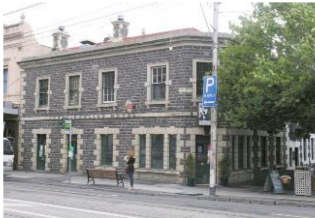
Figure 33. Grace Darling Hotel, Smith Street Collingwood (VHR H0660. Source: Victorian Heritage Database)
