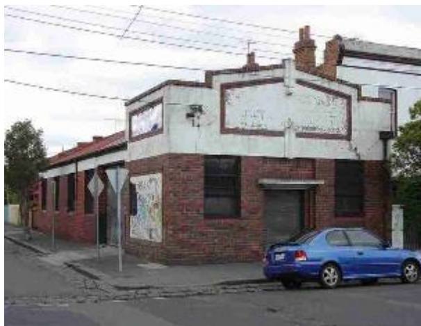
Figure 31. L.H. Lonsdale Motor engineering workshop at 12 Mater Street, Collingwood, Significant within HO321
