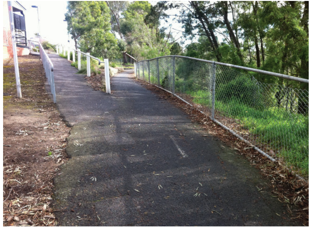
IMAGE 2 - LOOKING NORTH TOWARDS RUSHALL STATION
