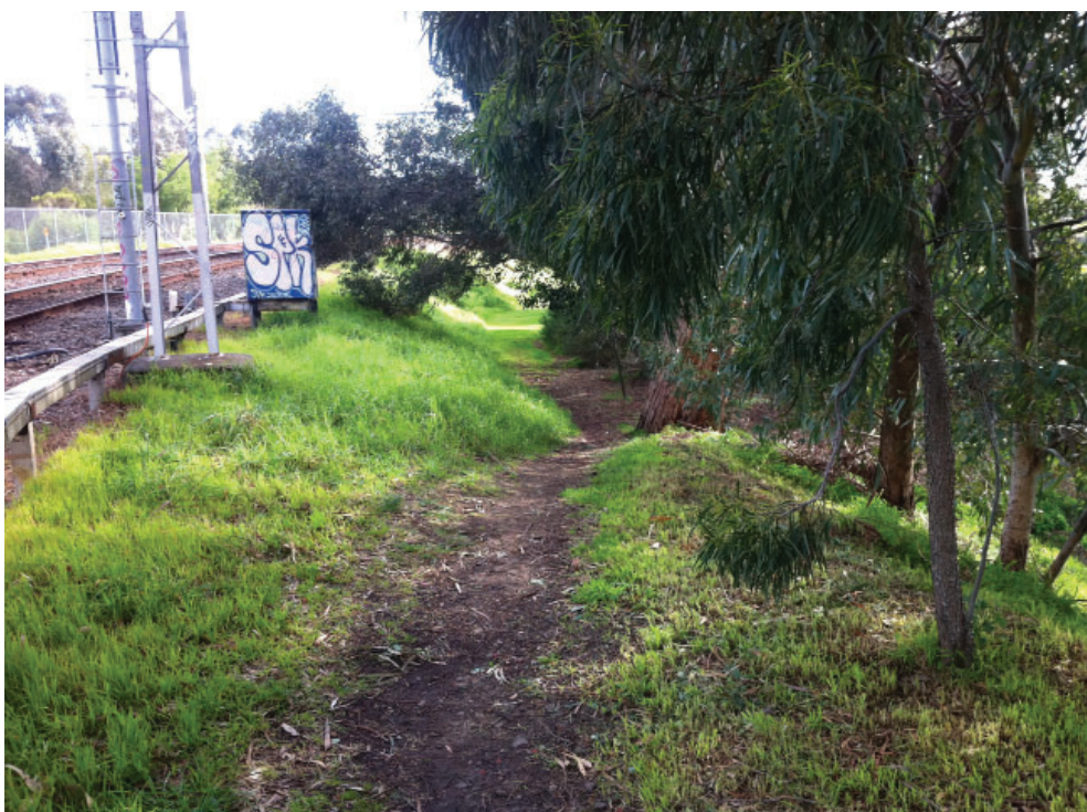
IMAGE 11 - STANCHION & SERVICE BOX
