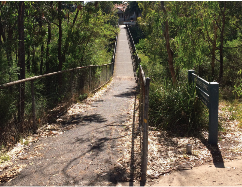
IMAGE 1 - BRIDGE TO NORTHCOTE 2M WIDE
