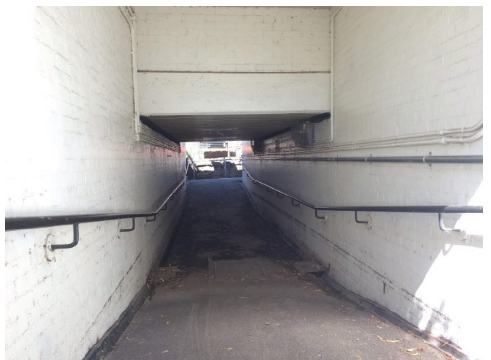
IMAGE 4 - EXISTING UNDERPASS - 2M WIDE - 2M HIGH
