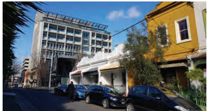
Views along Young Street toward ACU
