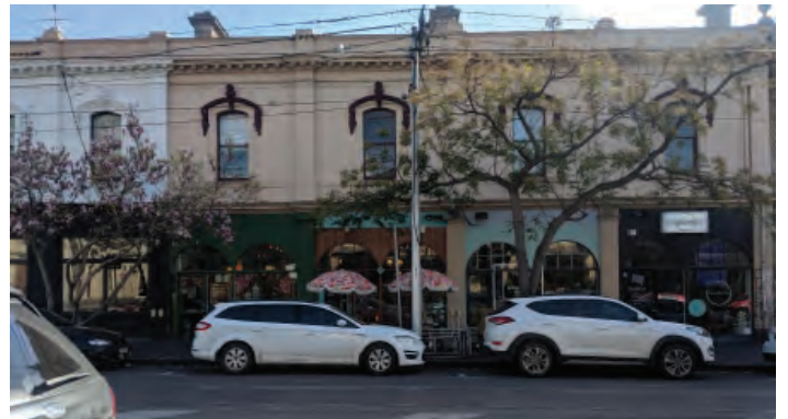
Orderly streetscape between Brunswick and Fitzroy Streets
