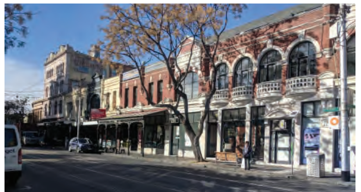
Buildings on the Gertrude Street crest, opposite Atherton Gardens
