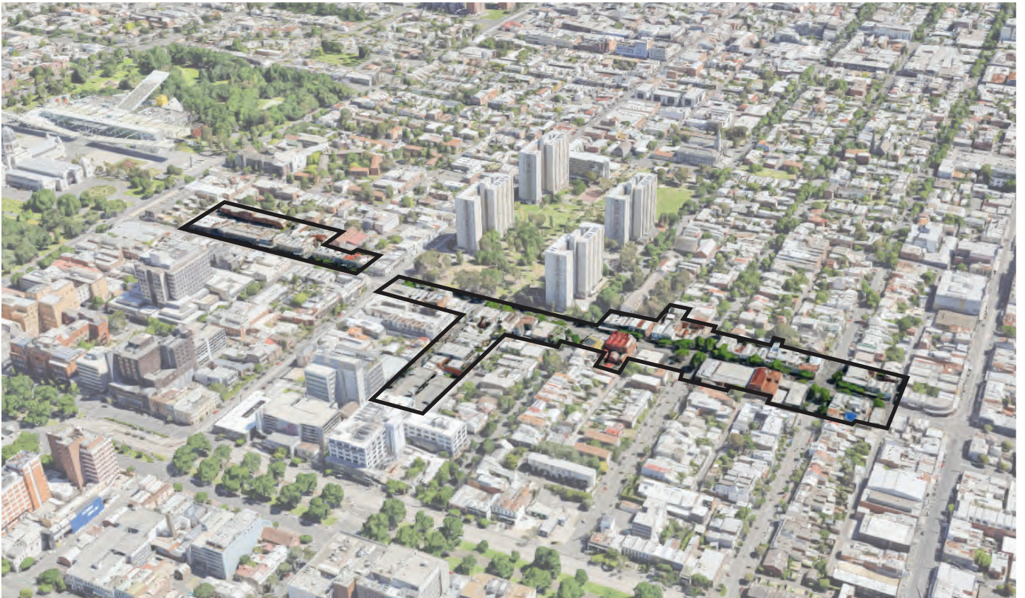
Oblique View of the Gertrude Street Study Area and Surrounding Context
