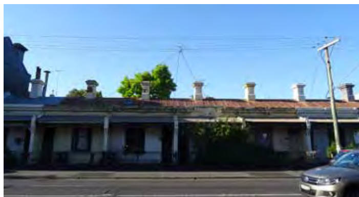
Row cottages along south side of Johnston Street, near Rochester Street
