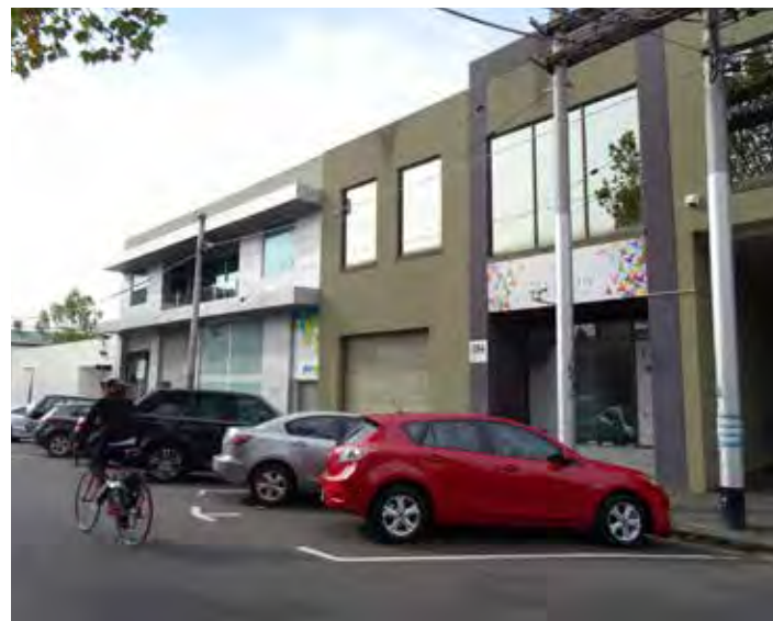
2 storey commercial forms on George Street
