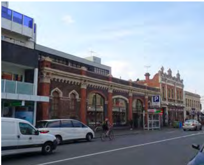
Heritage and non-heritage streetscape on the north side of Johnston Street
