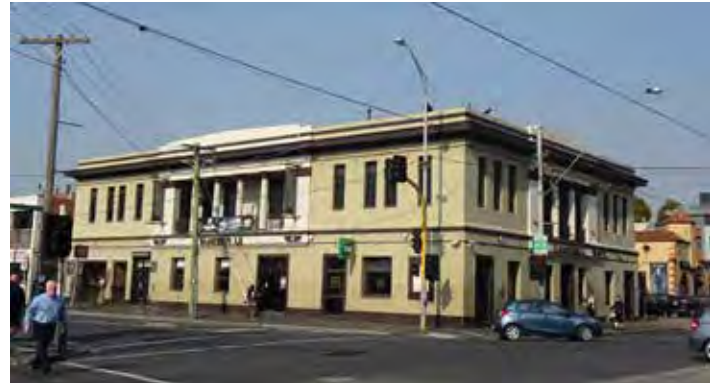
Tankerville Hotel, defines the corner of Johnston and Nicholson Streets
