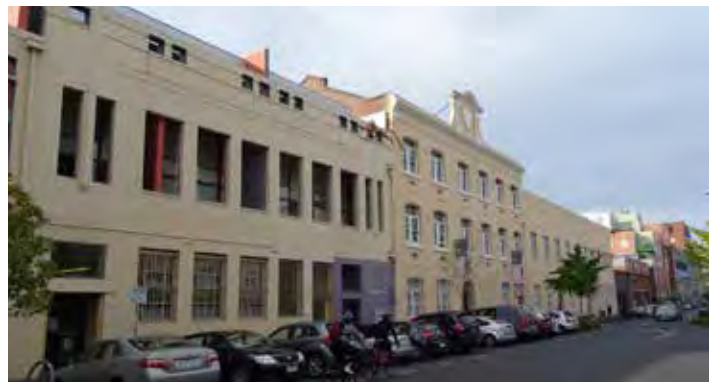
Former industrial forms along the northern side of Victoria Street
