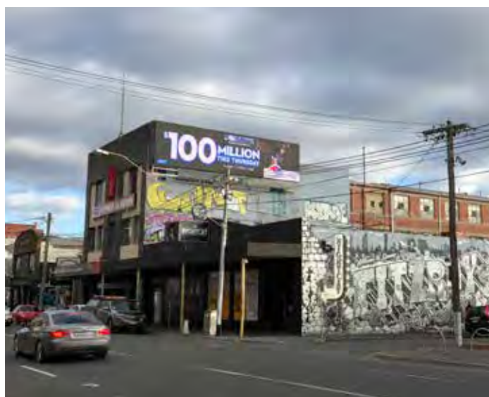
Non-heritage buildings on north side of Johnston Street, near Young Street
