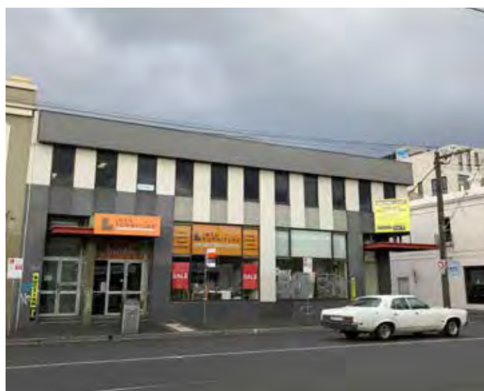
Non-heritage building on south side of Johnston Street, near Hertford Street
