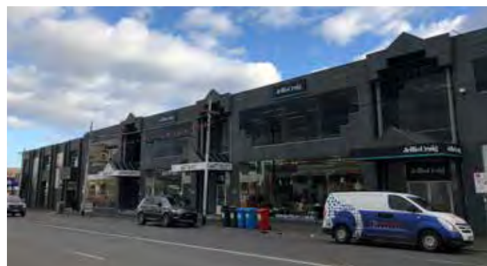
Non-heritage forms on the north side of Johnston Street (West)
