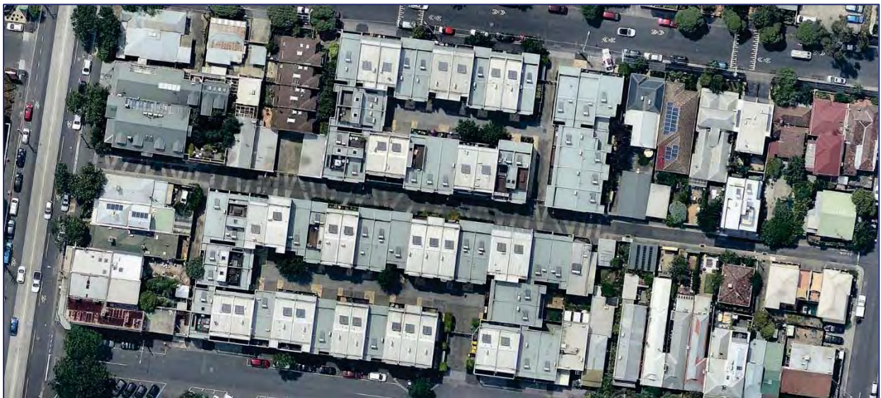
Figure 12: Shared Zone Example - Little Buckingham Street, Richmond
