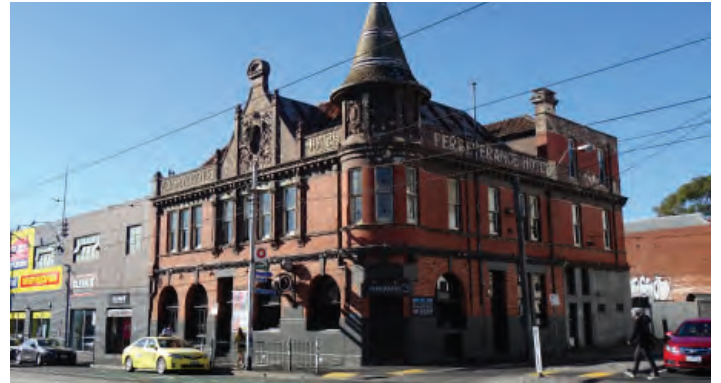
The Perseverance Hotel: local landmark at Moor and Brunswick Street
