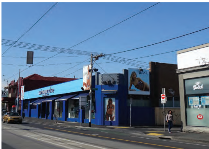
Example of a large, non-contributory site along the Brunswick Street spine
