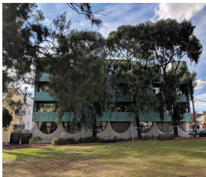
Recent development in Napier Street
