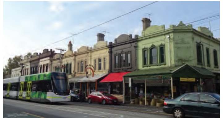
Consistent 2 storey street wall profile to the north of Johnston Street
