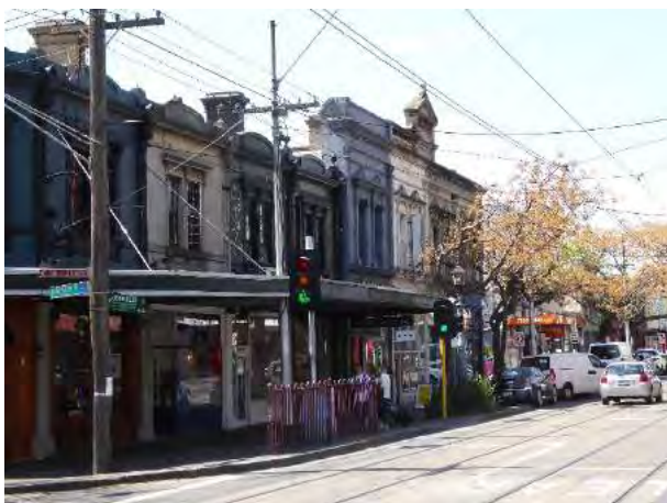
Figure 17. North side of Gertrude Street – east of Napier Street (GJM Heritage, October 2019)
