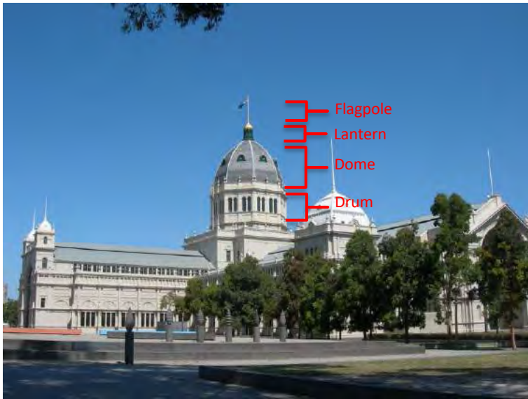
Figure 7. Royal Exhibition Building showing elements of the drum and dome (adapted from VHD, SOHE 2008)
