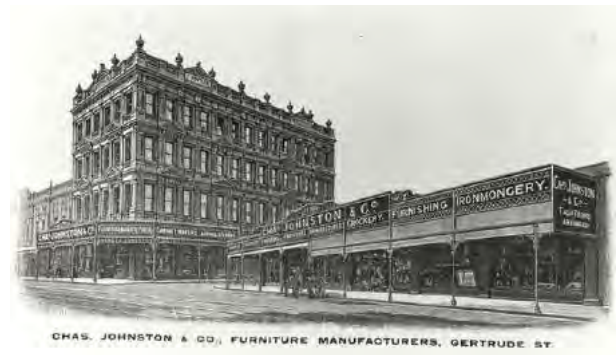
Figure 9. Illustration from the 1905 Collingwood and Fitzroy illustrated Directory and Handbook, of the multi-storeyed Chas. Johnston & Co., Furniture Manufacturers building at 184-186 Gertrude Street. The top two floors were destroyed by fire in 1963 (COYL, Id. FL670).
