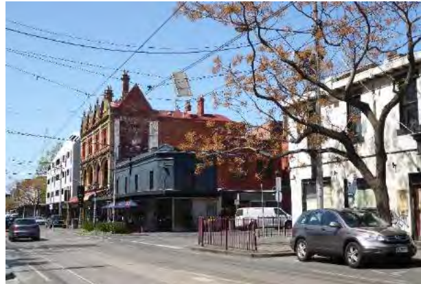
Figure 16. South side of Gertrude Street – eastern end (GJM Heritage, October 2019)
