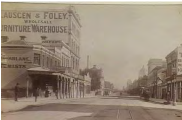
Figure 4. Looking west down Gertrude Street (from Young Street) towards the Royal Exhibition Buildings, c1890. The buildings on the right were later demolished to make way for the Atherton Gardens development (SLV, Image No. a13938).
