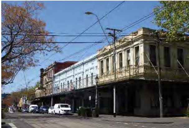
Figure 15. South side of Gertrude Street – east end (GJM Heritage, October 2019)
