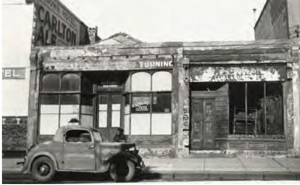
Figure 10. The poor condition of some shops in Gertrude Street in 1948 (COYL, Id. FL411).
