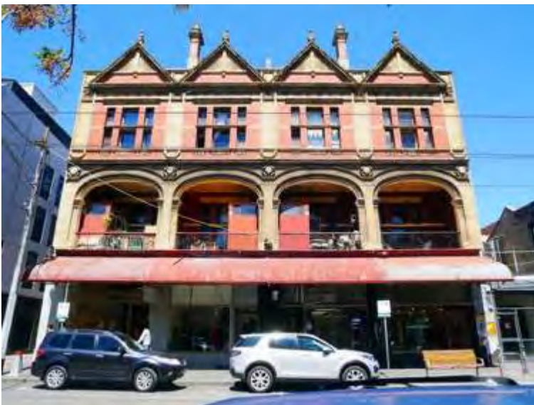
Figure 26. Blackett's Building at 158-164 Gertrude Street (at the intersection with Little George Street) is a freestanding tall, prominent and elaborately detailed three storey building with first floor loggia.
