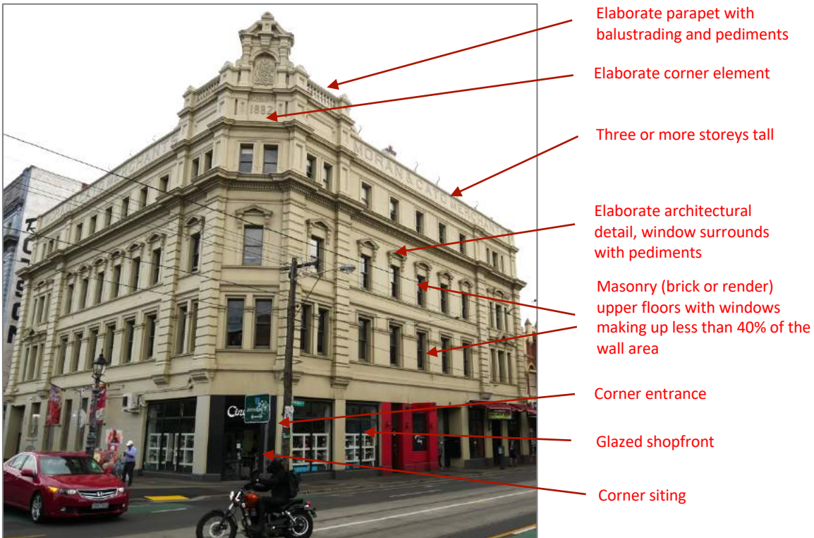
Figure 25. Department store / large commercial building (285 Brunswick Street)
