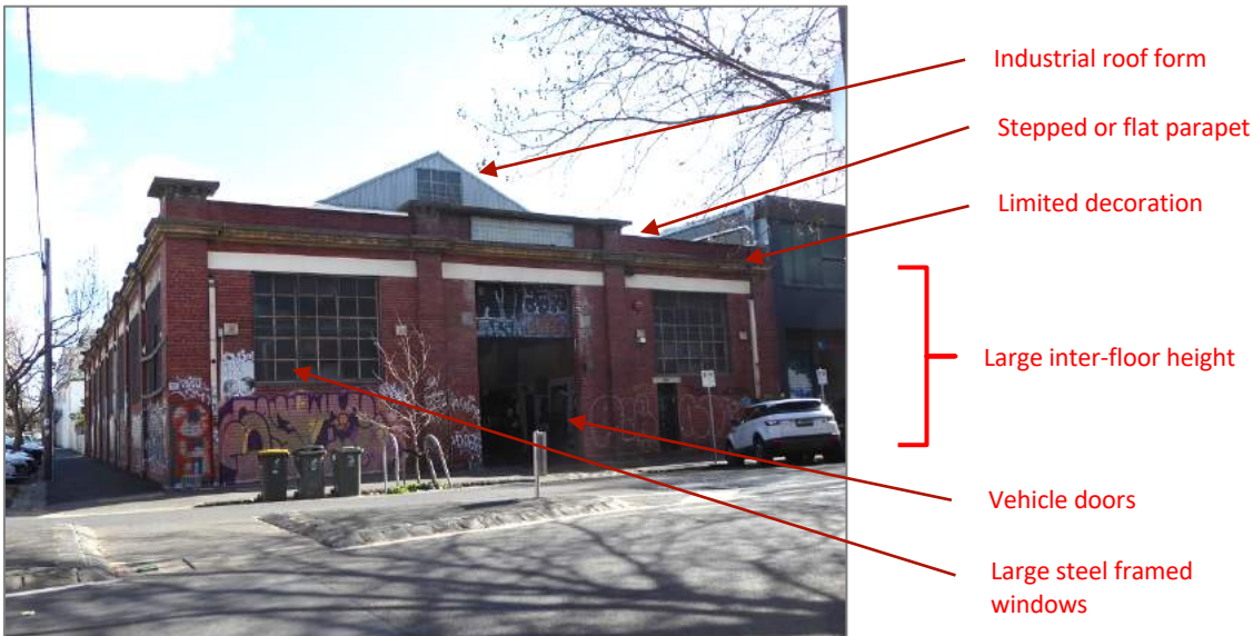
Figure 29. Low-rise (one to two storey) industrial buildings (399 Gore Street)
