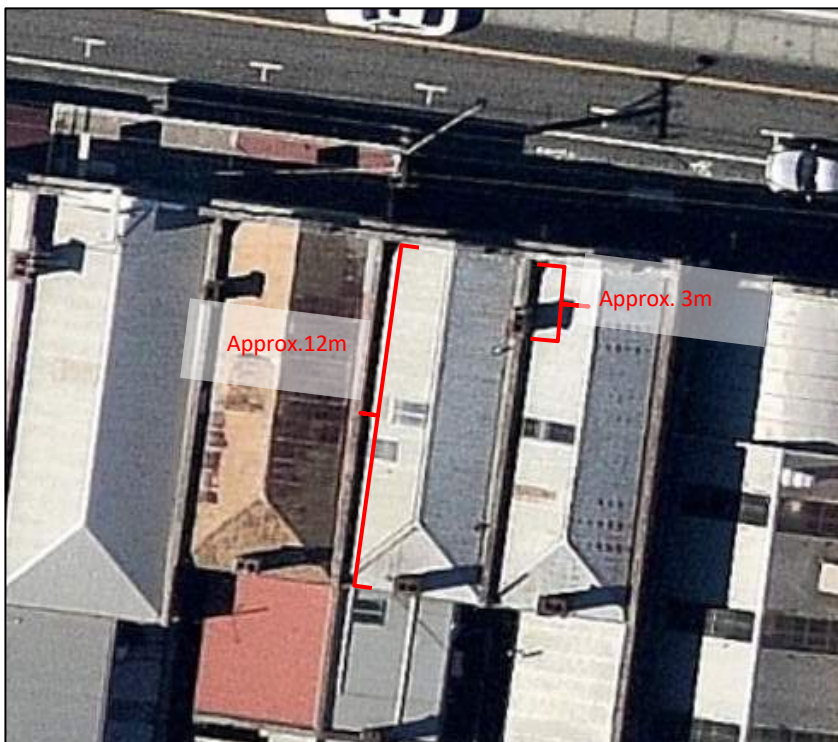
Figure 20. Roof plan (403-407 Brunswick Street, ©nearmap, 26 Sep 2017) showing the typical location of chimneys at the centre of each of the front rooms on the party wall (i.e. approx. 3m back from the front façade) and the typical 12m deep main roof form of the building.
