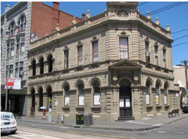
Figure 33. Former Union Bank of Australia, 165-167 Smith Street (VHR H0506) is an example of a local landmark due to its former use as a bank, its prominent corner location and elaborate architectural detailing (VHD, 2008)
