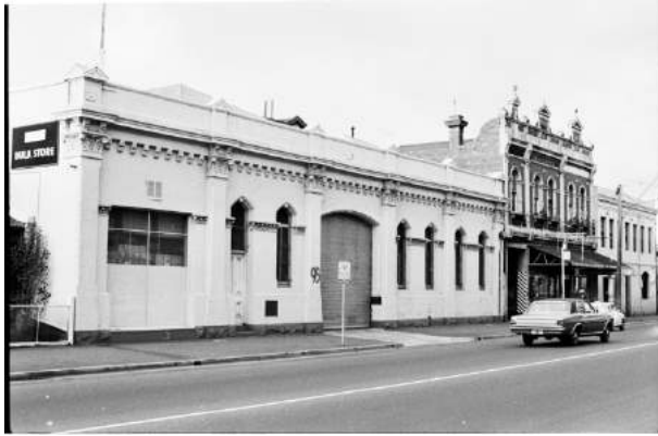
Figure 3. The Melbourne Tramway and Omnibus Co. tram engine house at 95 Johnston Street in 1970, prior to conversion to a supermarket (SLV, Image H2010.105/315b).
