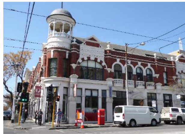
Figure 6. The Brunswick Street elevation (GJM Heritage, October 2019)
