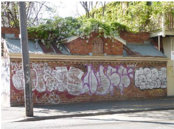
Figure 6. The remaining section of the gymnasium building (GJM Heritage, October 2019)
