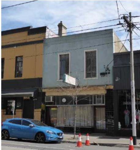
Figure 3. 131 Brunswick Street, Fitzroy (GJM Heritage, Oct 2019)
