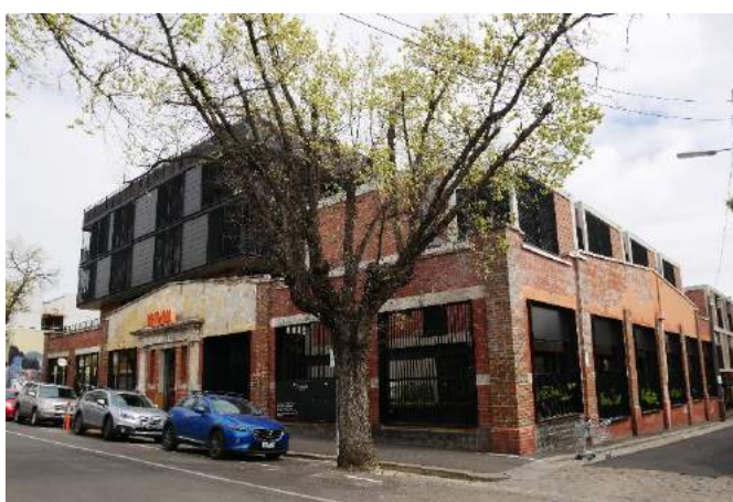
Figure 26. 237-241 Napier Street, Fitzroy. Top: St David Street and Napier Street elevations. Bottom: Napier Street and Exhibition Street elevations (GJM Heritage, Oct 2018)
