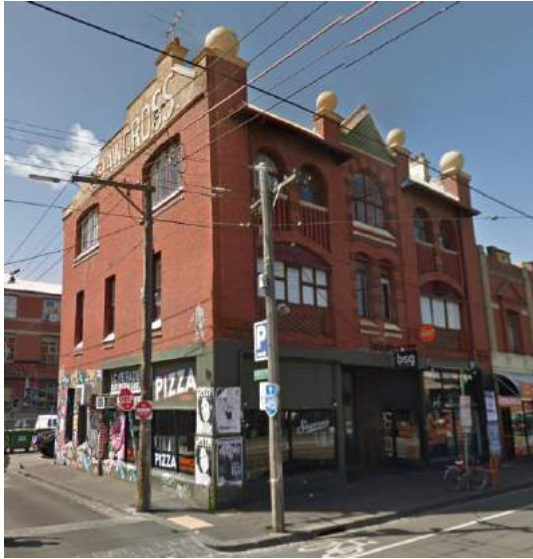
Figure 16. Shawcross Building, 320 Brunswick Street, Fitzroy (Google)
