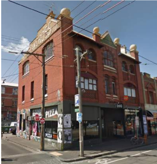
Figure 10. Shawcross Building, 320 Brunswick Street, Fitzroy (Google)
