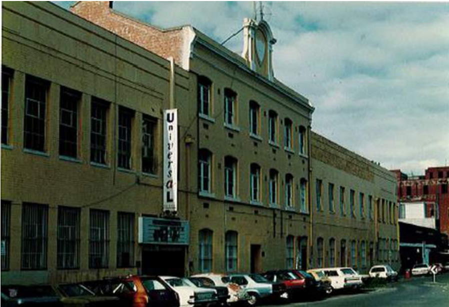
Figure 62. The former Acme shirt factory and La Mode Corset factory on Victoria Street, Fitzroy, in the late twentieth century (Past Port, 'ACME Shirt Factory/La Mode Corset Factory, 31-39 Victoria Street', < https://pastport.com.au/citizen/record/660/ >, accessed 7 Aug 2019).
