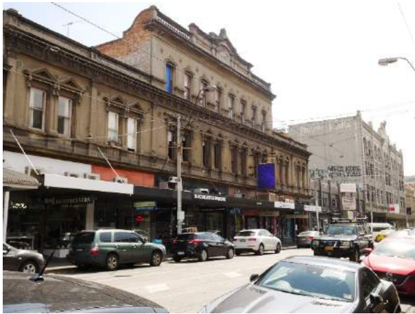
Figure 25. Stanford Block, 119-29 Smith Street, Fitzroy (GJM Heritage, Sep 2017)
