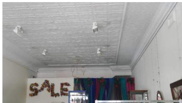
Figure 72. Interior of 61 Smith Street (Oct 2018)
