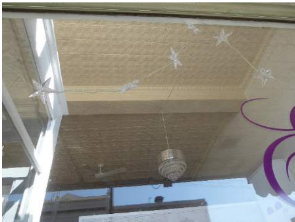
Figure 32. Interior of 51 Smith Street (Oct 2019)
