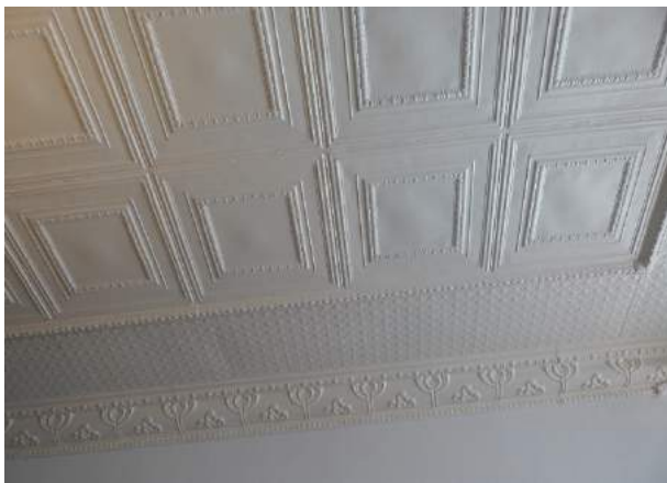
Figure 39. Interior of 67 Smith Street (Oct 2019)
