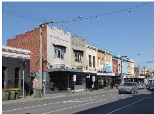
Figure 13. South side of Johnston Street, west of Smith Street (GJM Heritage, October 2019)
