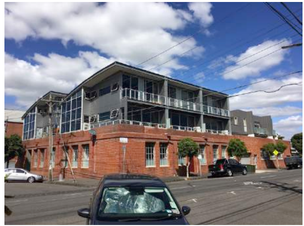
Figure 53. 98-100 Roseneath Street, Clifton Hill (GJM Heritage)
