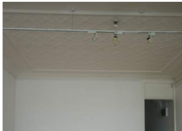
Figure 40. Interior of 69 Smith Street (Oct 2018)
