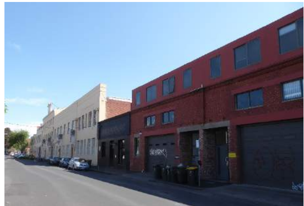
Figure 17. North side of Victoria Street – left is the La Mode Corset Factory complex at the west end (GJM Heritage, October 2019)
