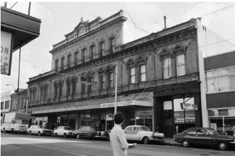
Figure 4. Stanford Block in 1970 (SLV, Image No. CUAFY48/1-3).
