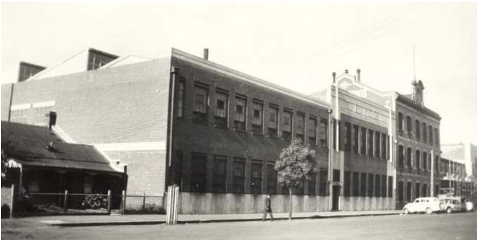
Figure 60. 'La Mode Corset Industries' on Victoria Street; photo taken in 1948. The three-storey building was originally the Acme Shirt Factory (City of Yarra Libraries, ID No. FL464).
