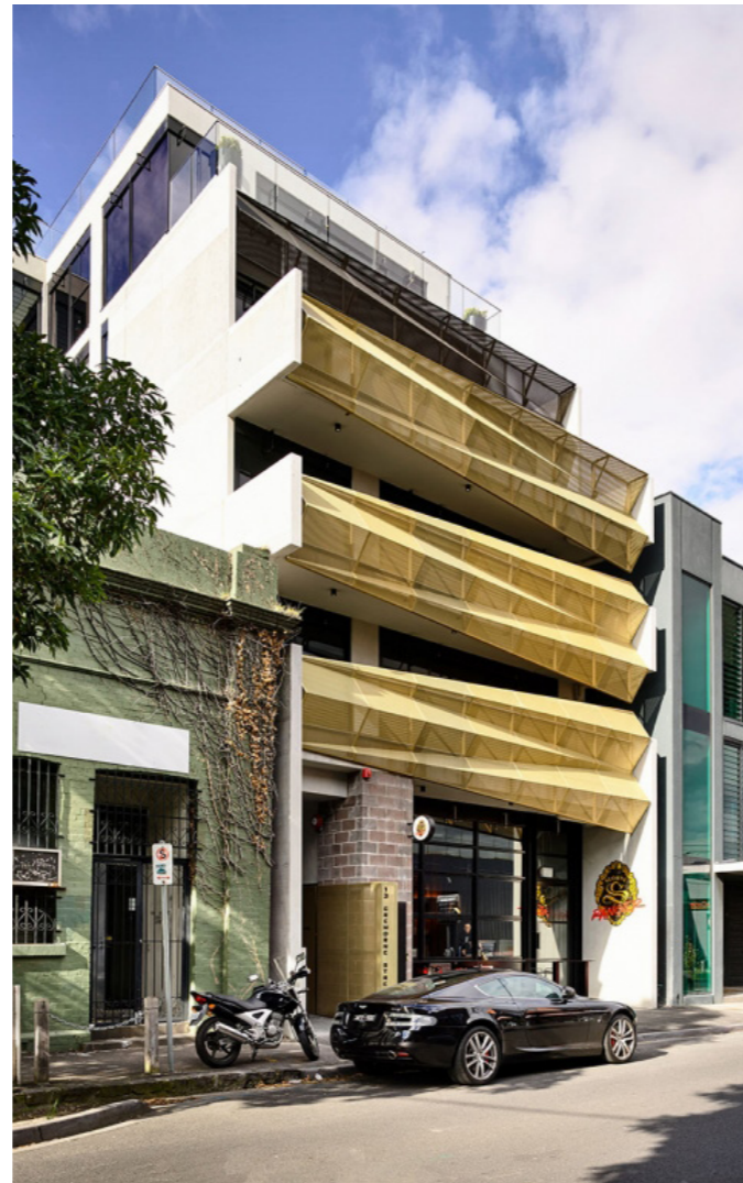
Figure 79. Commercial development in Cremorne (Source: EAT Architects)
