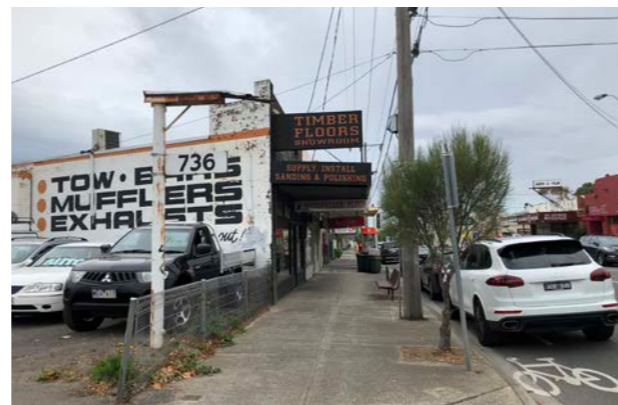
Figure 5. Example of poor street activation - at grade car parks front directly onto street.
