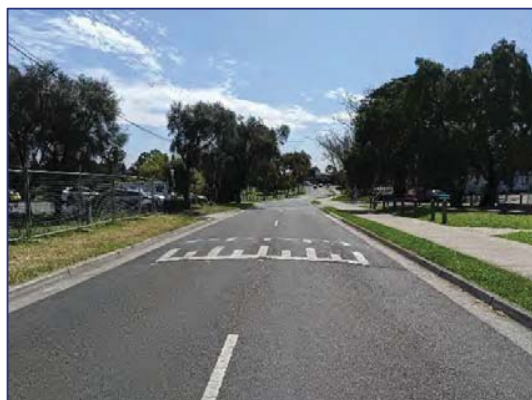
Figure 13: Yarra Bend Road - view north
