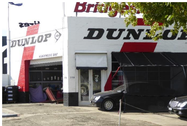
Service centre – west elevation
