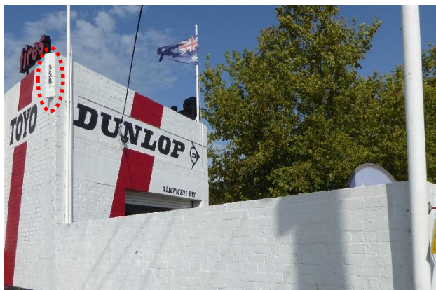
Service centre – north-east corner elevation Note 'tires' signage mounted to parapet and small projection with street number (highlighted)
