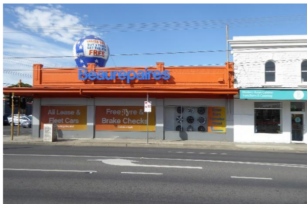
Heidelberg Road (north) elevation
