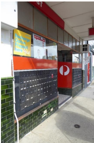
No. 730 Heidelberg Road – typical Interwar shopfront configuration
