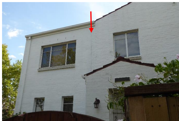
House – south elevation, window openings and portico. The junction between the original eastern section and later west wing is evident.
