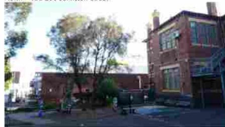
South – Fitzroy Primary School – looking towards site
