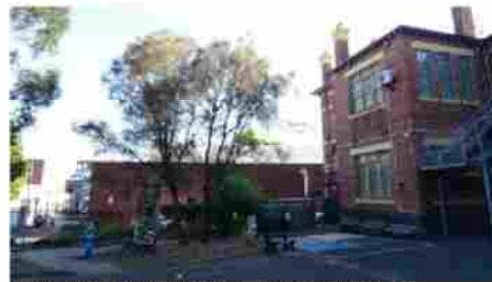
South – Fitzroy Primary School – looking towards site
