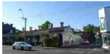
North – 188-200 Johnston Street
