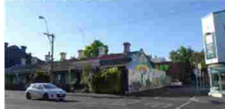
North – 188-200 Johnston Street
