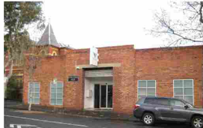
Current George Street Facade of Existing Building
