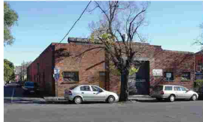
George Street facade prior to alterations circa 2005/6. Source: Victorian Heritage Database © City of Yarra
