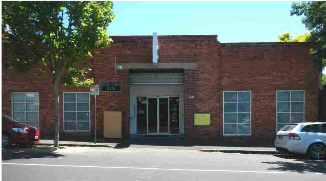
The building has been further altered from the above photo principally by the removal of the roof lantern and the long windows in the façade.
