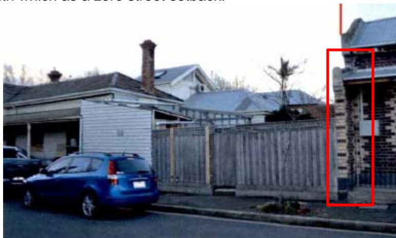
Figure 2: Western boundary wall of No. 96 Yarra Street (Applicant Submission)
