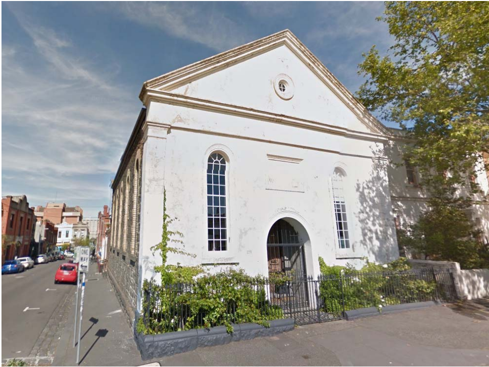
Gore Street facade
