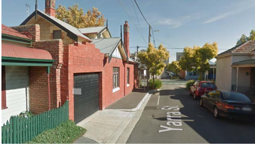
Figure 8: View of No. 194 Nicholson Street (Google Maps)
