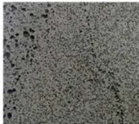
Diamond-sawn Bluestone paving - Bamstone (street interface)
