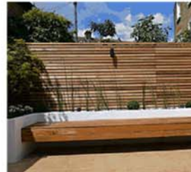
Concrete planter box with inbuilt timber seating elements.
