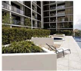
Concrete raised planter with contrasting textures, such as vegetation, decking and stone unit paving.
