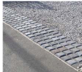
Porphyry stone rumble strip to driveway areas
