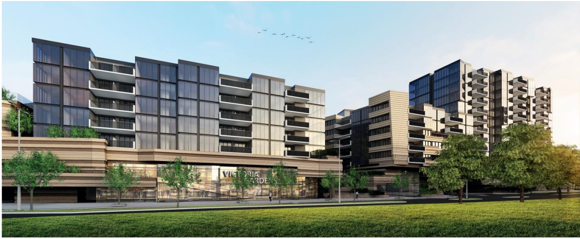
View looking West across River Boulevard
