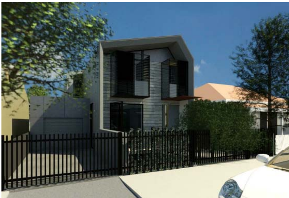
Render of the proposed dwelling with the garage material modified to sheeted zinc to match the dwelling
