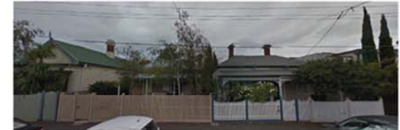
STREETVIEW TOWARDS DWELLINGS 17 & 19 GREEN ST.
