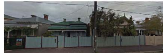
STREETVIEW TOWARDS DWELLINGS 13 & 15 GREEN ST.
