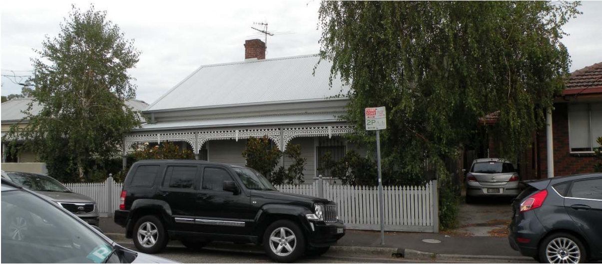
Above: Adjacent Individually significant property at no. 16 Green Street
