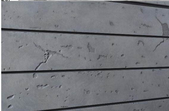
Above: Examples of concrete walls with horizontal joint lines
