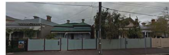
STREETVIEW TOWARDS DWELLINGS 13 & 15 GREEN ST.
