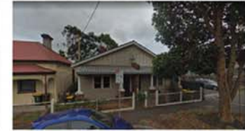
STREETVIEW TOWARDS DWELLINGS 8 & 6 GREEN ST.
