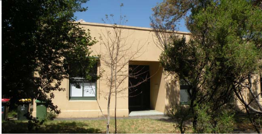
Above: View towards subject site from Church Street
