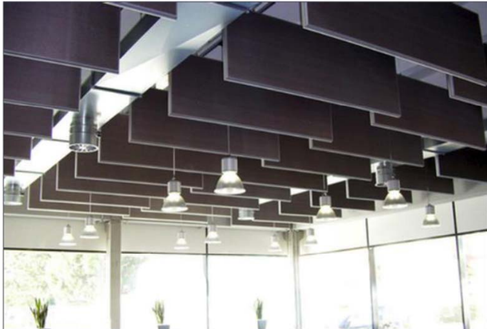
Figure 7: Baffles hung from the ceiling.
