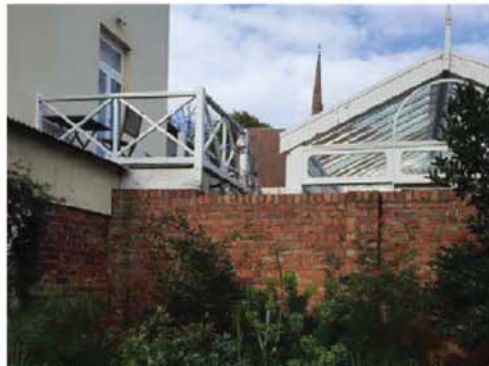
10 VIEW FROM BACKYARD TO No. 14 REAR 1:7.14
