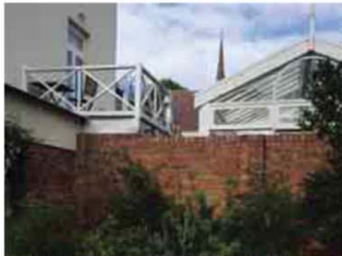
10 VIEW FROM BACKYARD TO No. 14 REAR 1:7.14
