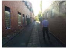
DOVE PLACE FACING WINDOWS (LEFT - 88 TYPE ST, RIGHT - 84 TYPE ST) TRANSLUCENT GLASS BLOCK WINDOWS
