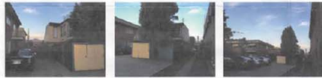
REAR OF 84 TYPE STREET (ADJACENT TO 76 TYPE STREET CARPARK - LEFT) REAR OF 84 TYPE STREET (BE TWEEN 76 TYPE STREET CARPARK ON LEFT & DOVE PLACE ON RIGHT) DOVE PLACE (FACING TOWARDS TYPE STREET)
