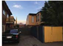
REAR OF 84 TYPE STREET (ADJACENT TO 76 TYPE STREET CARPARK - LEFT)
