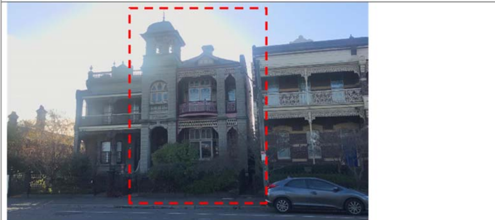
Above: View towards subject site from immediately across Alfred Crescent.
