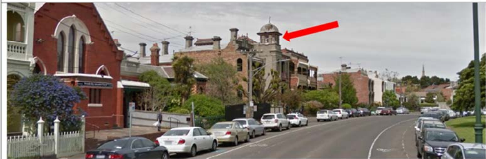
Above: View towards subject site from the far south-west.
