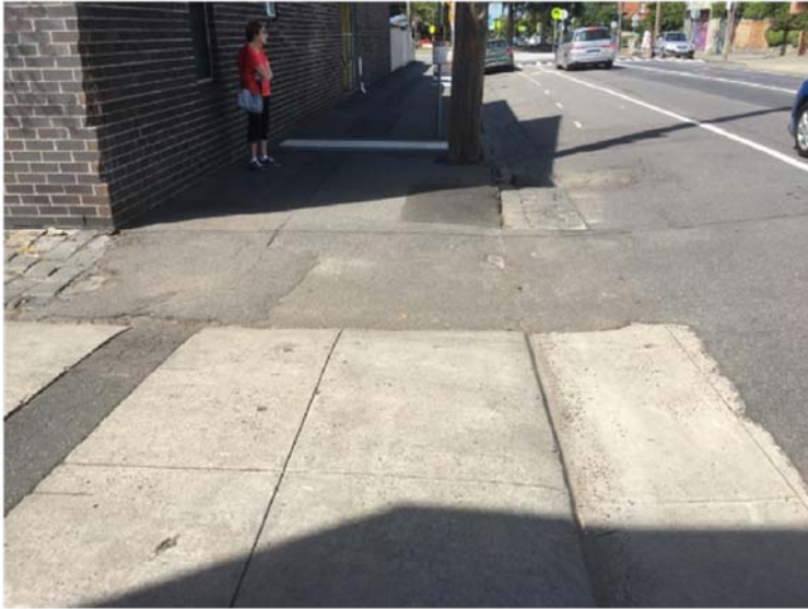
Existing vehicle crossing servicing the Right of Way and development site.
