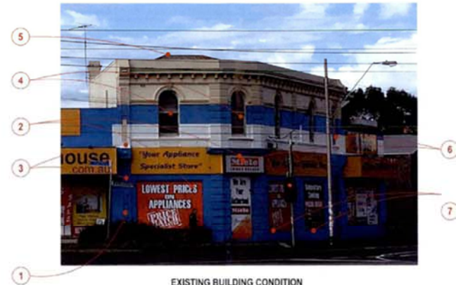
EXISTING BUILDING CONDITION
