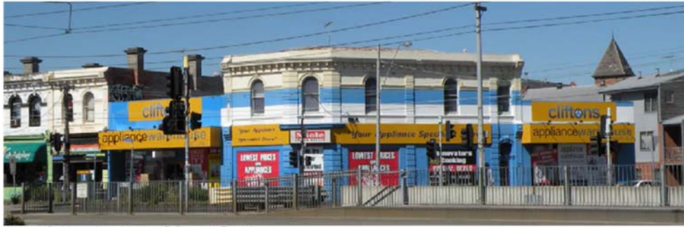
Above: Subject site at 141-147 Queens Parade
