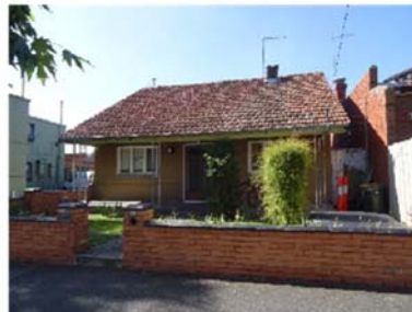
View of residential property directly north of the site
