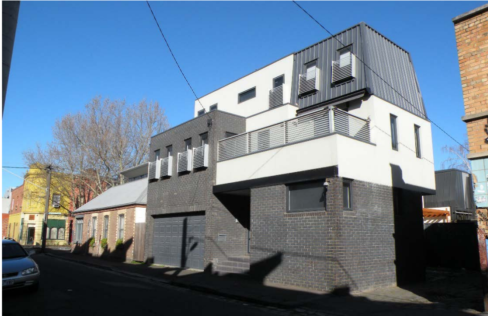
Above: Development directly behind the subject site fronting Fitzroy Street (No. 467 Fitzroy Street)
