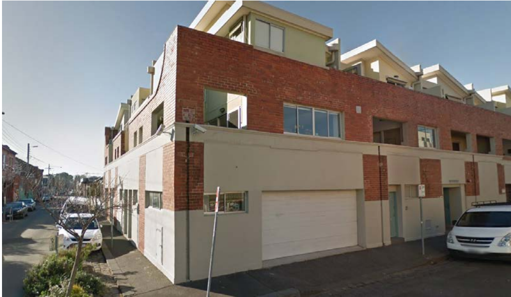
No. 498 Fitzroy Street (east)
