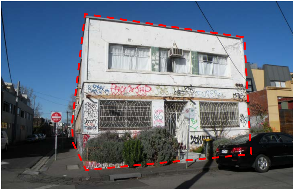
Above: Subject site as seen from across the street
